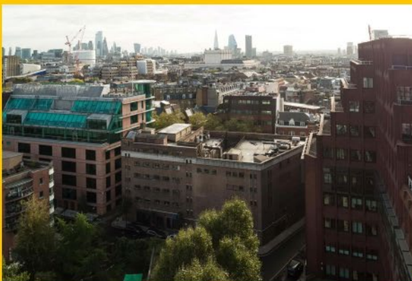
135 Shaftesbury Avenue Rear View
