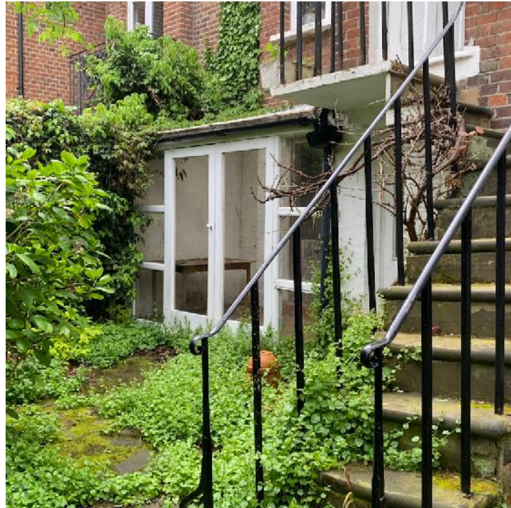
Existing Conservatory – extremely inefficient construction
