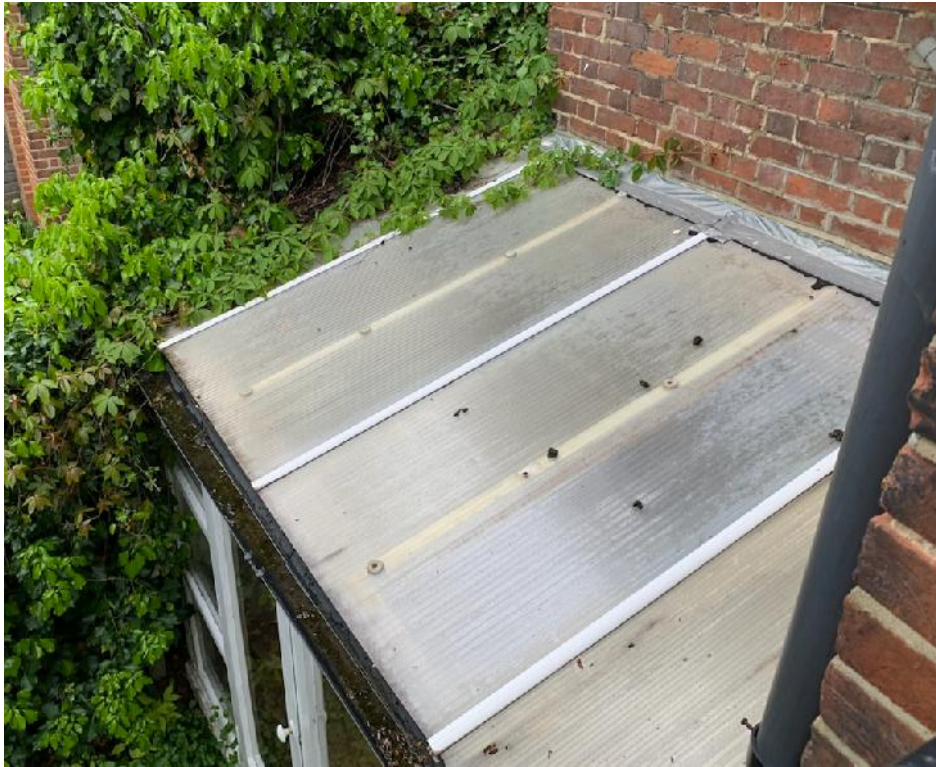
Existing Conservatory Roof
