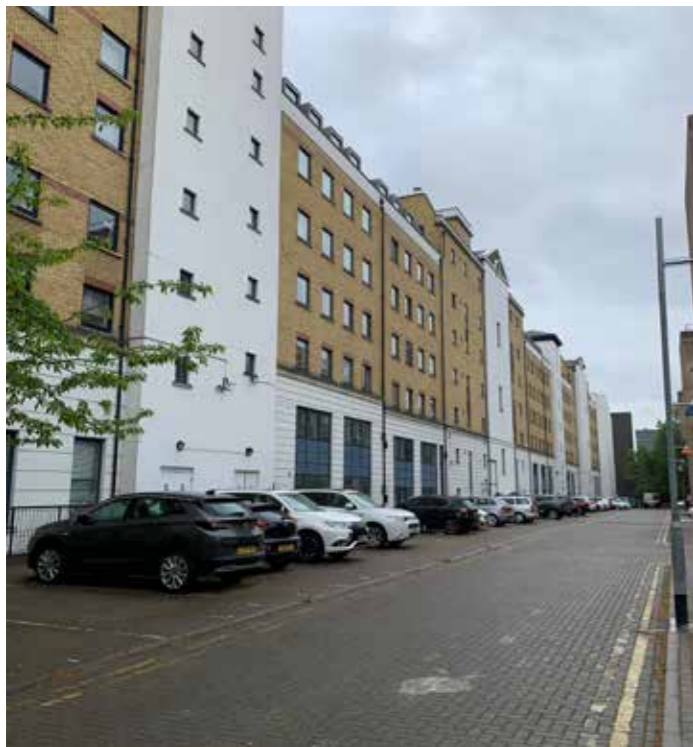
Figure 3.16 Rear elevation. View looking from the north
