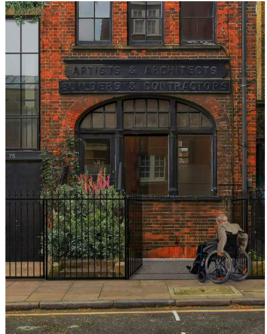
Fig. 4. The renovated building provides step-free access
