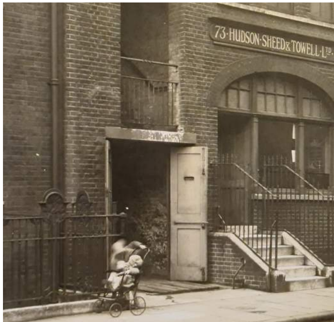
Fig. 8. Original Door at 73-75 Kenton Street
