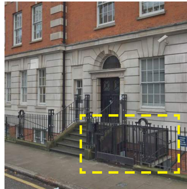
Fig. 16. 38 Bidborough Street with external platform lift
