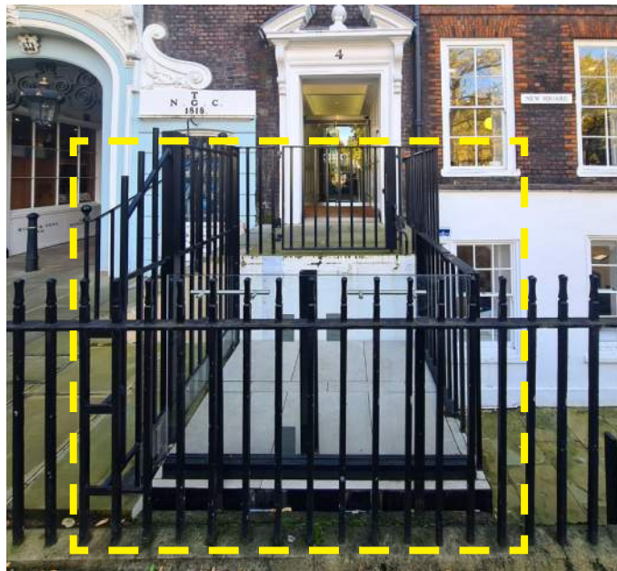
Fig. 15. 1 New Square with external platform lift
