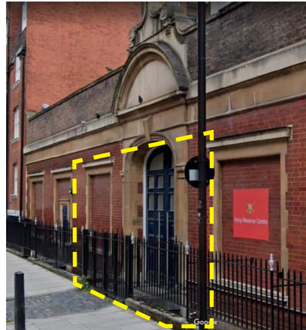
Fig. 9. Army Reserve Centre, with concrete plinths and metal swing gates
