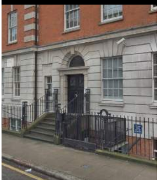
Lightwell lift - Bidborough St.
