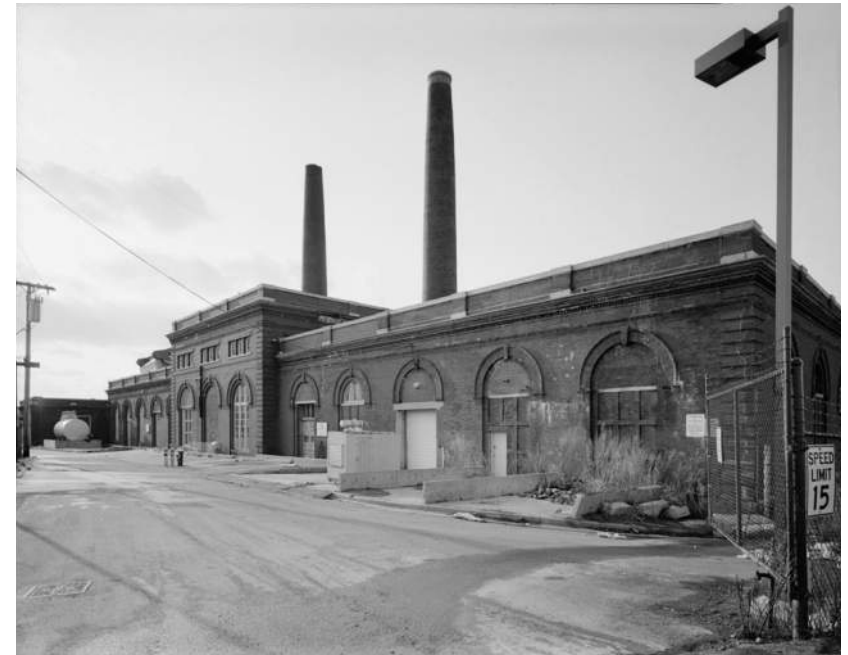
Fig. 1. Preservation and energy upgrade of Pump House in East Boston, MA, USA
