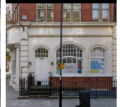
Gated steps - Hastings St.
