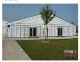
The Alu Hall is supplied with rigid PVC sidewall panels. The roof of the structure will be supplied in opaque (non-permeable to light) high grade PVC. The Neptunus rain gutter tensioning system ensures that the roof canopy stays taut at all times and rainwater is drained at central points. The structure will be installed with a raised and self-weighted cassette floor system that protects the existing hard standing.
