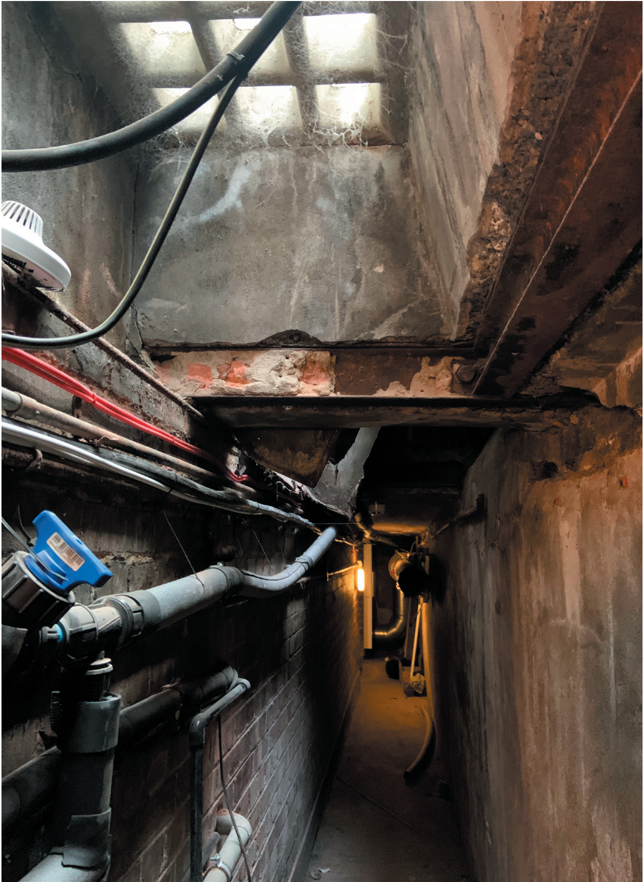
Photo of one of the existing West Street passage where the existing steels show visible signs of corrosion and delamination.
