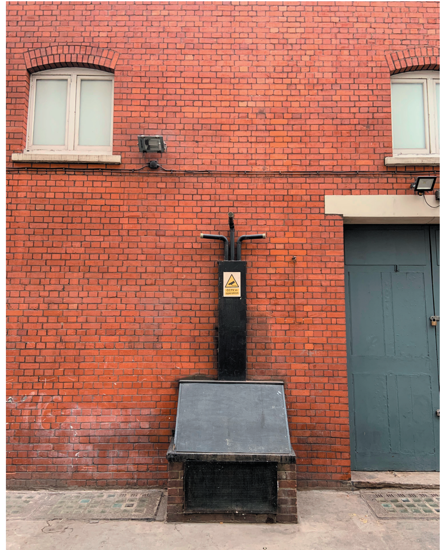
Photo of the existing redundant pipework proposed for removal on Tower Court side
