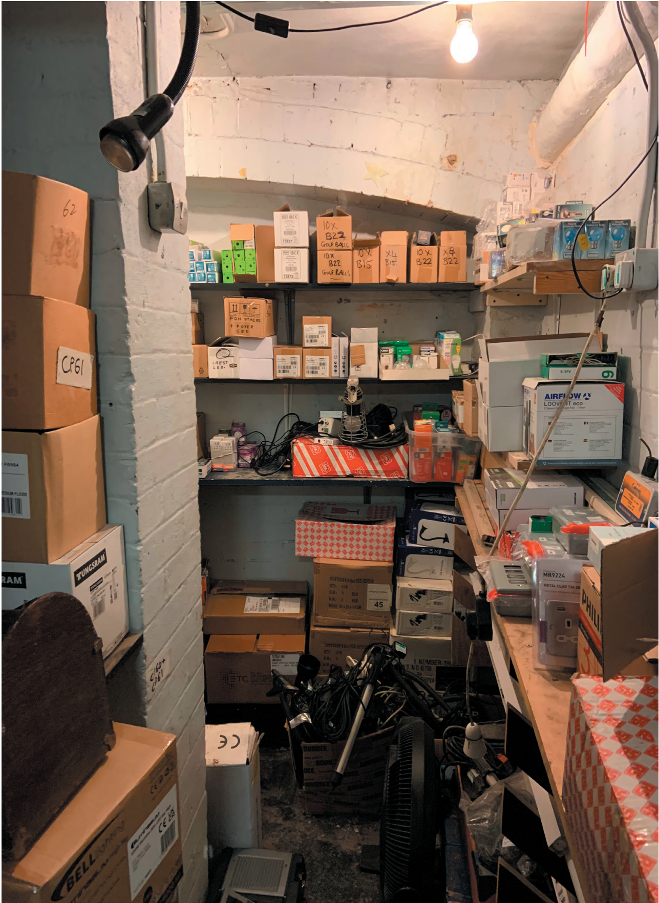
Photo of the existing masonry arch at sub-stage level where it is proposed to form the new fire escape route
