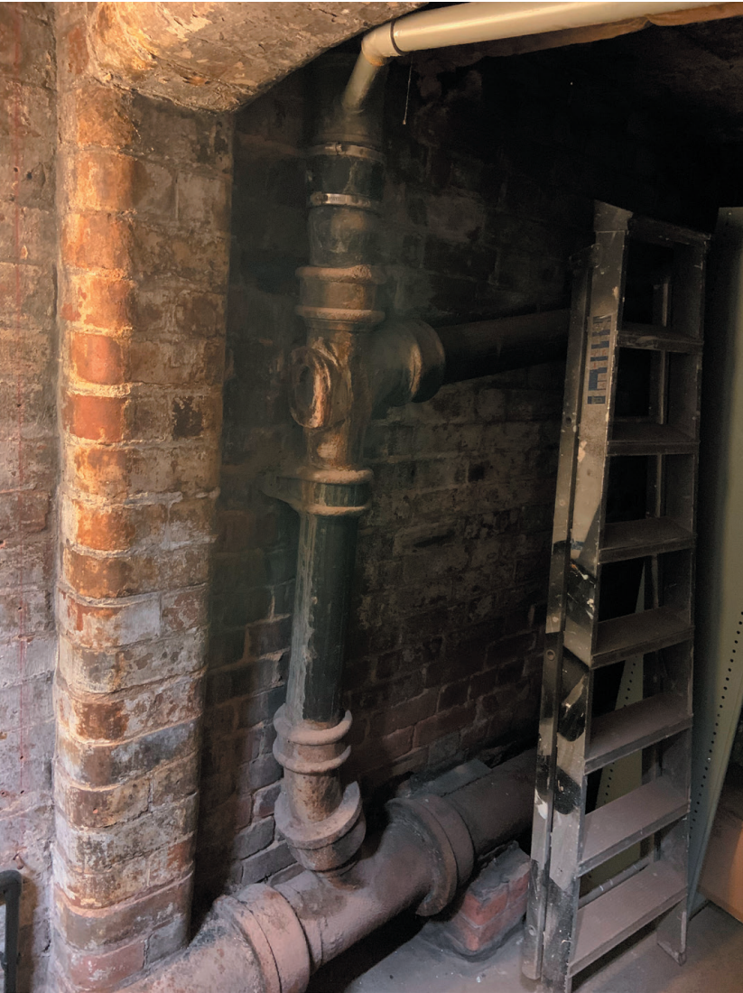
Photo of the existing masonry wall at sub-stage level within the existing Boiler Room where it is proposed to form the new fire escape route
