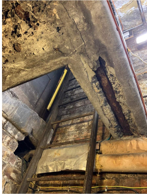
Left photo: small portion of the boiler room floor seen from stalls level. Right photo: existing structure seen from below, showing the significant corrosion and subsequent spalling of the concrete.
