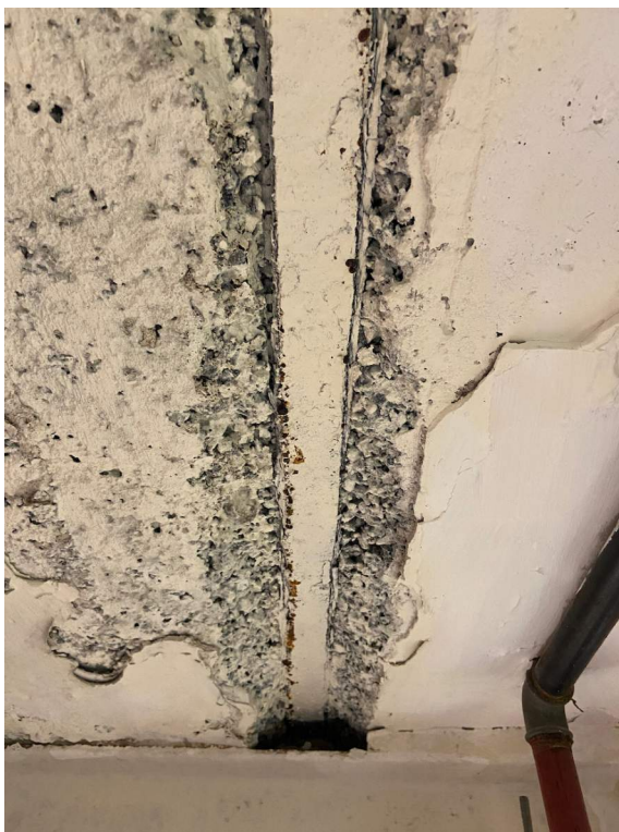
Left photo: the concrete encasing around the bottom flange had spalled, due to corrosion expansion. Right photo: the corrosion was quite severe in certain locations, with delamination of the steel.
