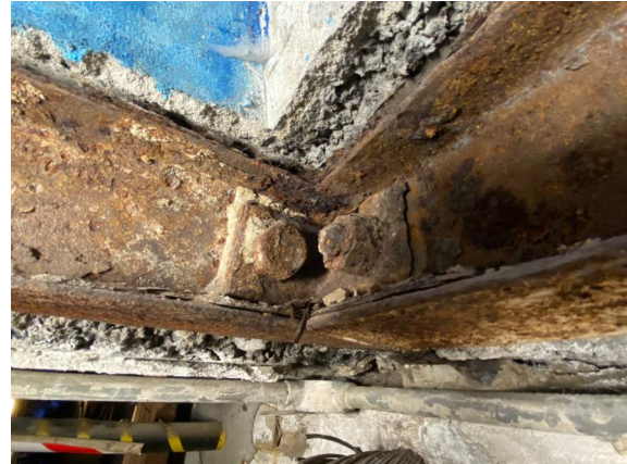
Left photo: the concrete encasing around the trimming steel beams had spalled, due to corrosion expansion. Right photo: delamination was severe in certain locations, in particular on the top and bottom flange.
