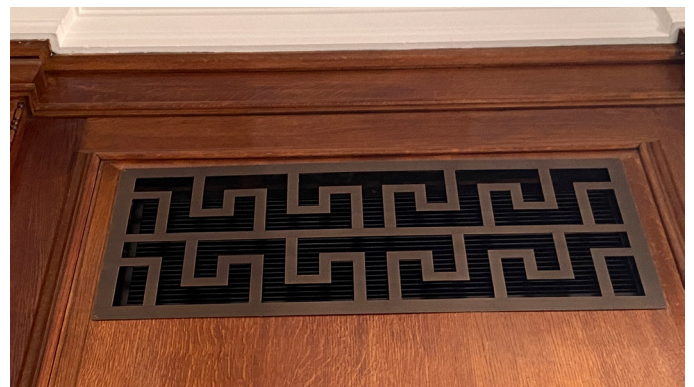
New patinated brass ventilation grille to the first floor democratic spaces
