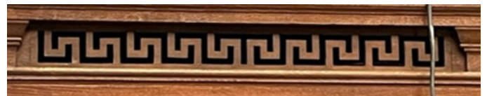
Existing Council Chamber timber ventilation grille
