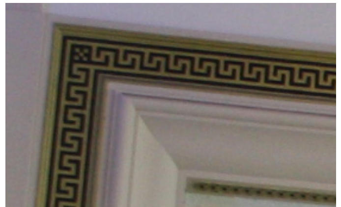
Existing Camden Centre timber decorative facade
