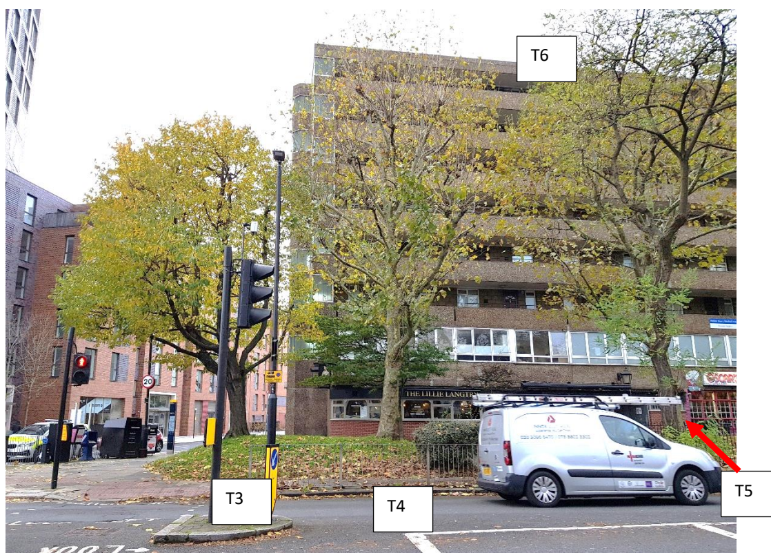
Photo 1 of T3, T4 and T6 looking south. November 2019.
