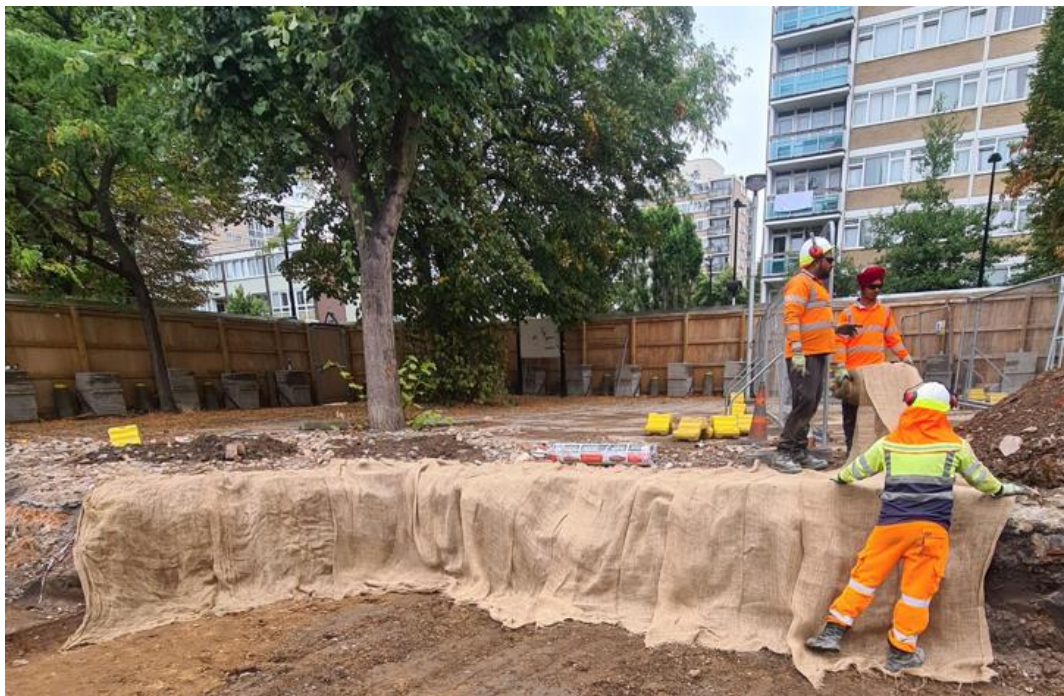
Photo 6 taken of a different site supervised by SHA after root pruning, and showing hessian
