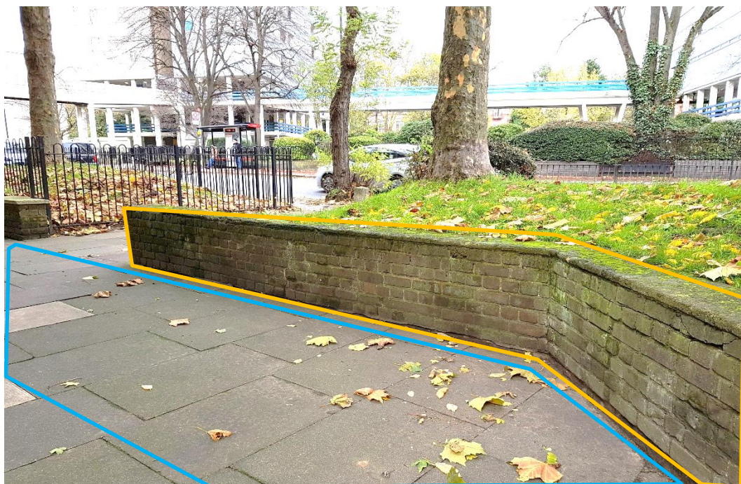
Photo 8. Paving to be retained during demolition and construction and removed during the external works phase as shown by blue line on the photo and brown hatching on the plan
