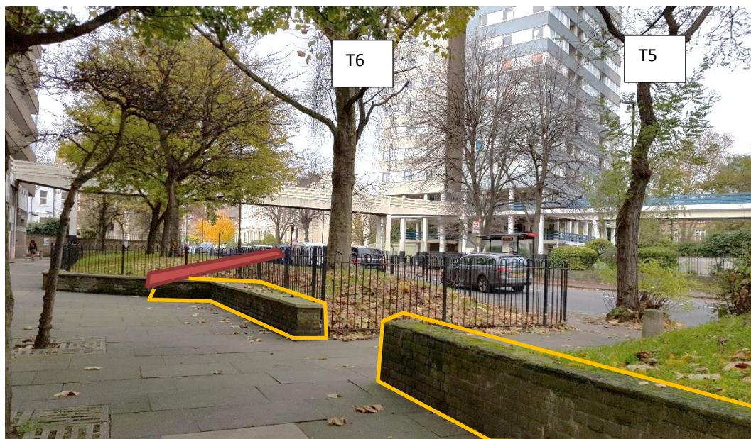
Photo 4 of T6 looking north east. Area for excavation shown red. Retained walls shown yellow.
