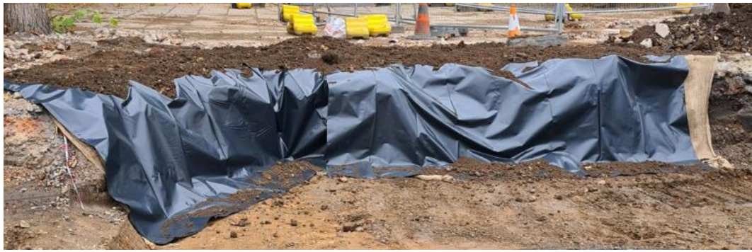
Photo 7 taken of a different site supervised by SHA after root pruning, and showing plastic sheeting weighted with soil. The piling mat will be installed up to this point and the tree protection fencing will be reinstated along the line.
