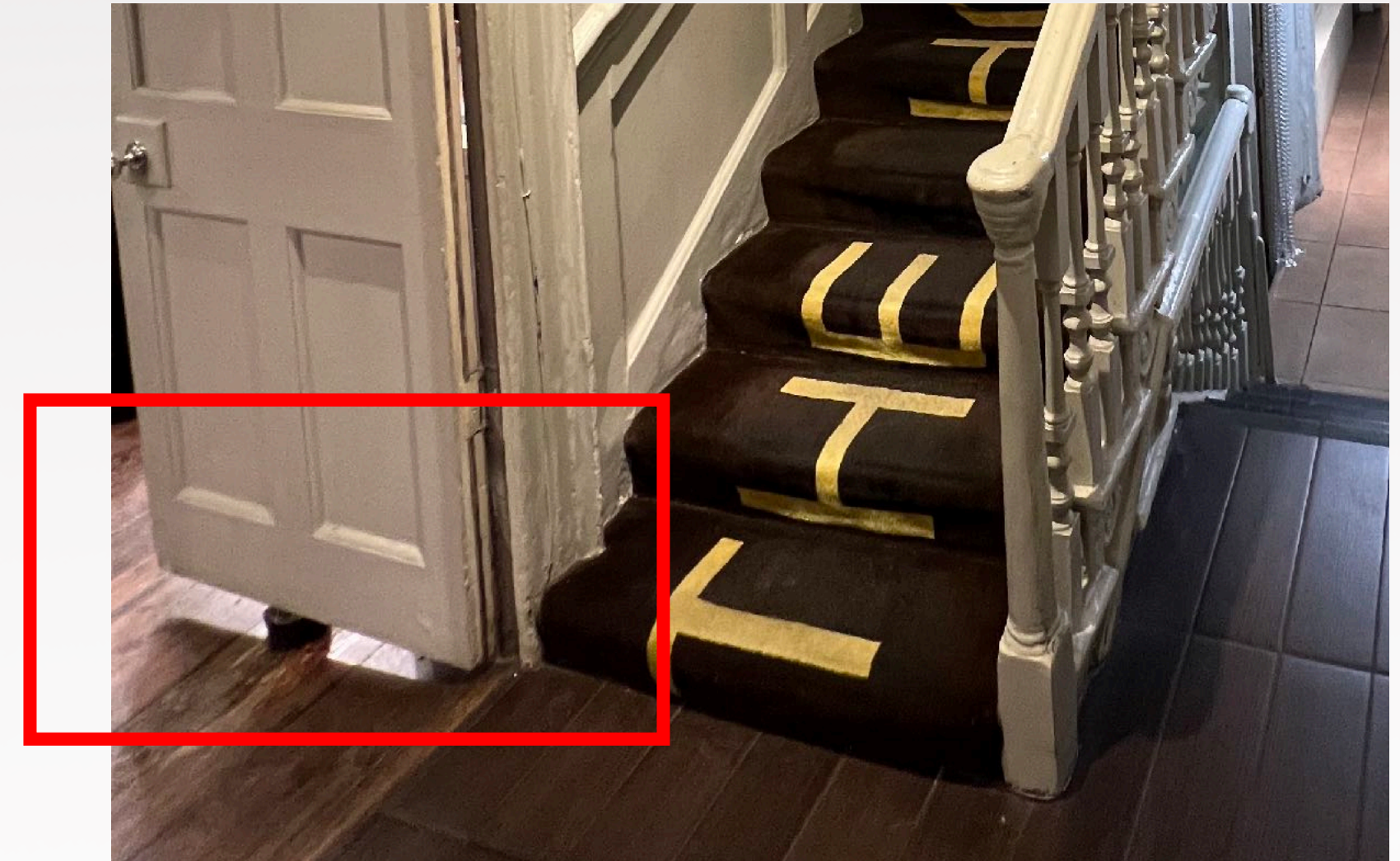
Typical gap at foot of 'fire doors'
