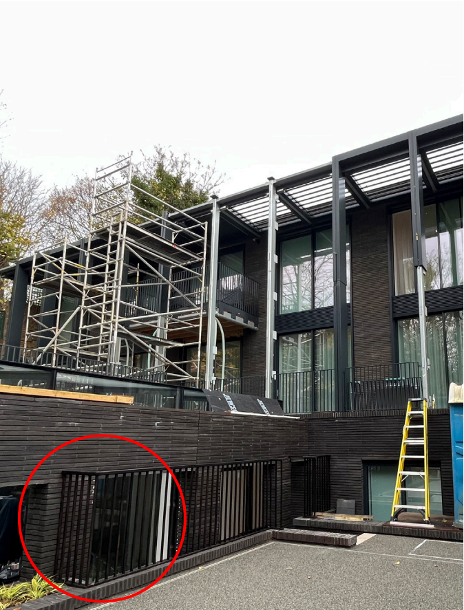
Current condition A temporary timber balustrade has been installed, which will be replaced by the proposed external metal balustrade. To be powder coated to match the existing metal balustrades.
