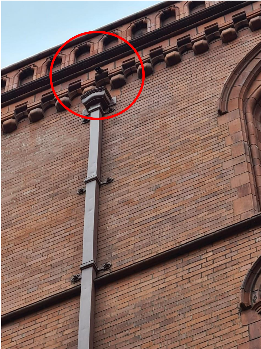
Existing overflow chute to be replicated under this proposal.
