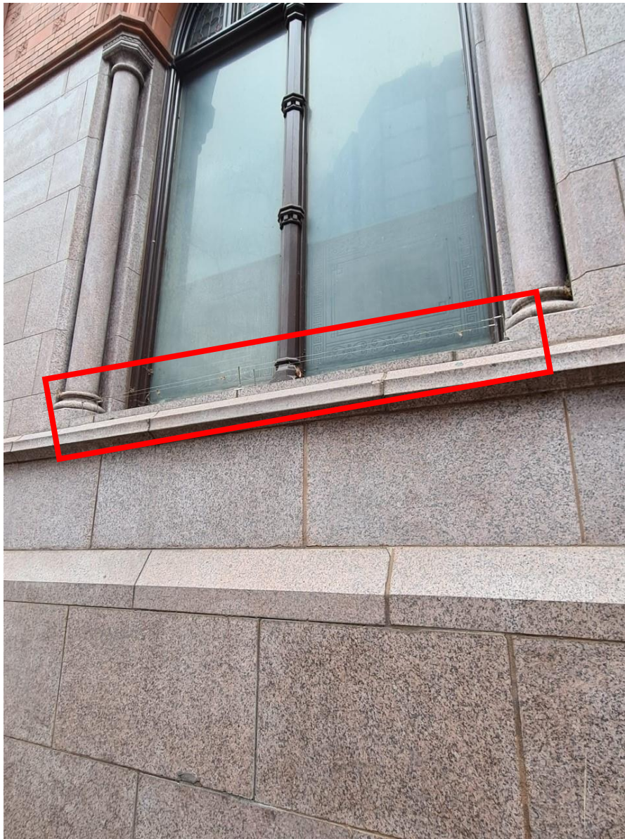
Existing pigeon wire installation to be replicated under this proposal.
