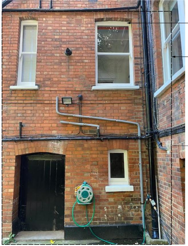
Existing Ground floor \_window to laundry room Proposal is to extend window opening to fit new door to access stair.
