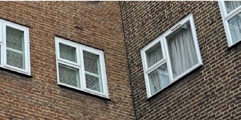
Fig 23. The existing elevation with the dual toned brickwork skin.
