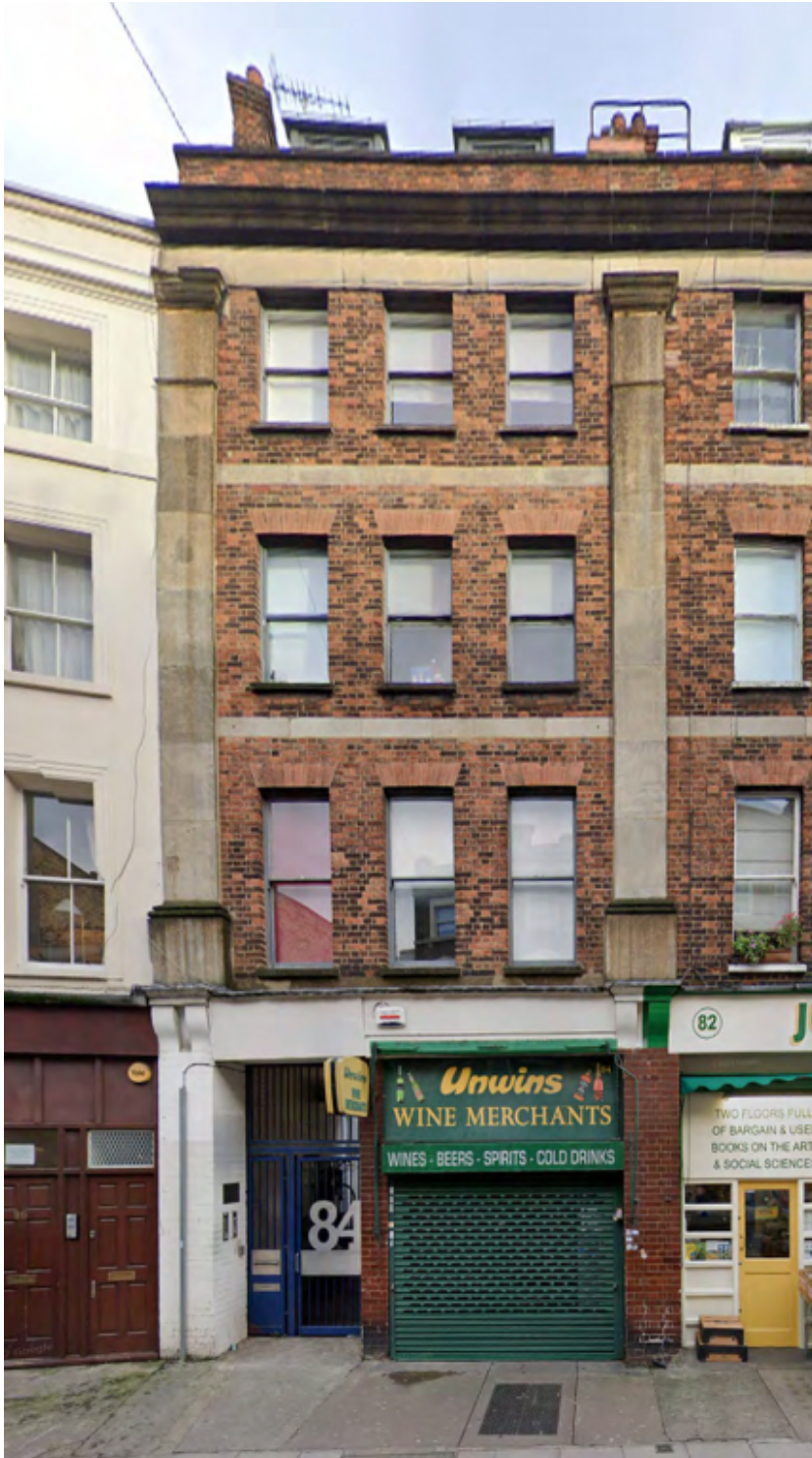
Photo 1 (above): View of existing shopfront with roller shutter closed
