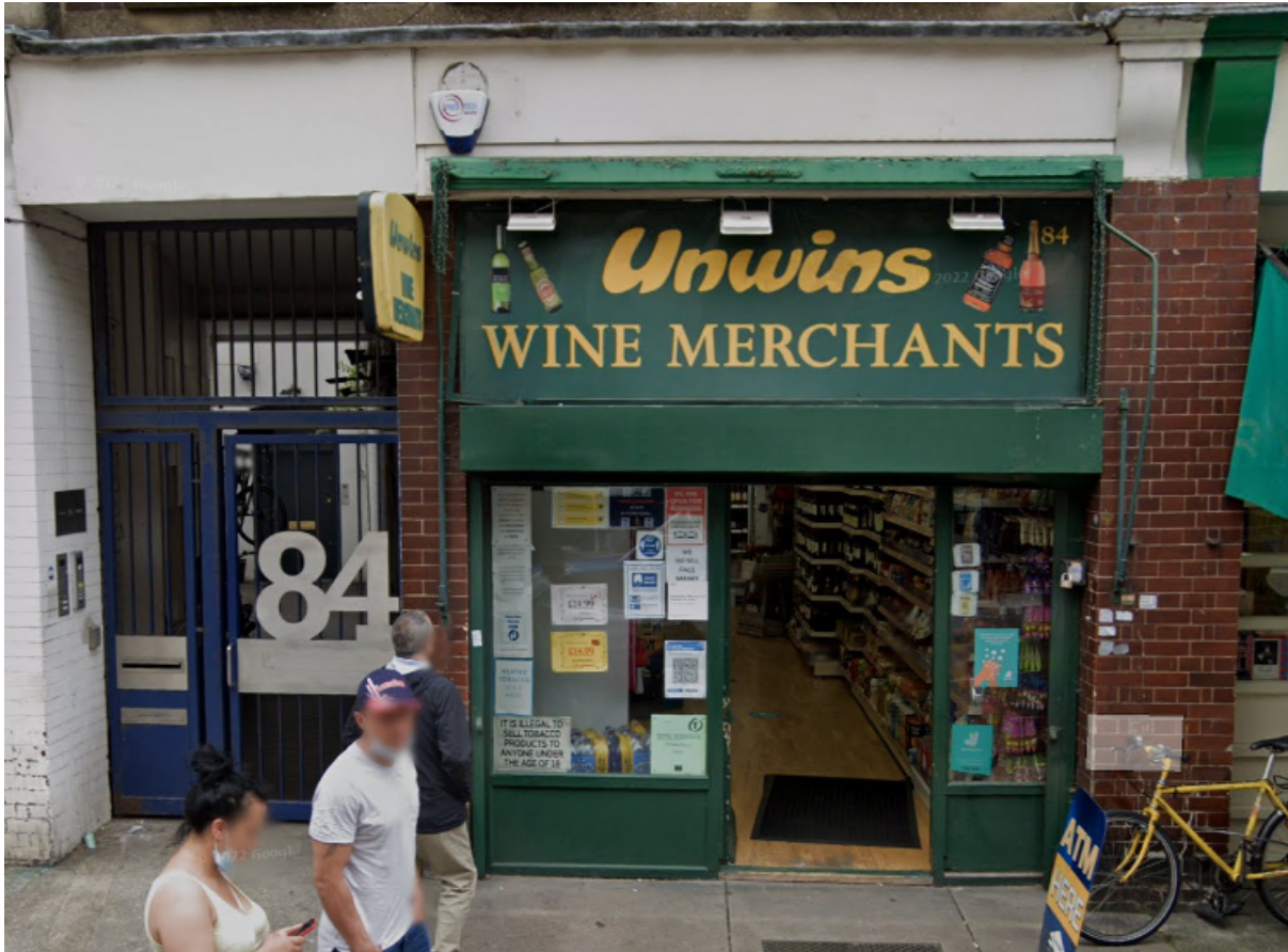
Photo 2 (above): Close-up view of existing shopfront with roller shutter open
