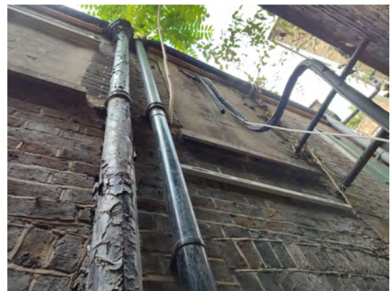
Blocked up ground floor window 2 (from basement courtyard)
