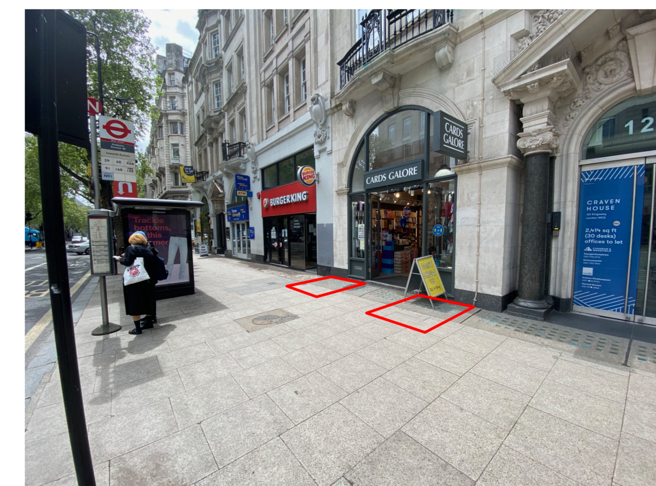
2 PHOTO OF PAVEMENT AREA TO FRONT OF RETAIL UNIT (HISTORIC) NOT TO SCALE
