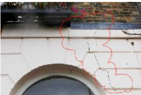
Photo 2 : Above Front Entrance. Refer dwg. nos. JGPS/CHAR/4/5/100RevA, 5016334/RDG/XX/XX/DT/S/0200Rev.T3 and 5016334/RDG/XX/XX/EL/S/0300Rev.T3
