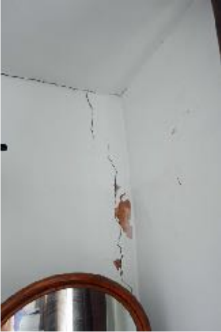
Photo 9 : Second Floor. Refer dwg. nos. JGPS/CHAR/4/5/101RevA, 5016334/RDG/XX/XX/DT/S/0201Rev.T3
