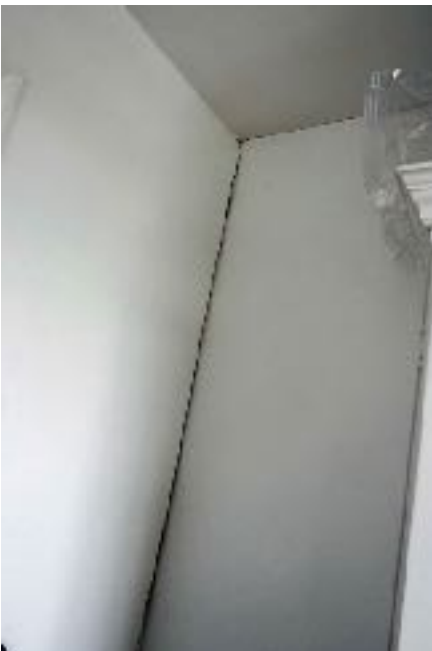
Photo 7: Second Floor. Refer dwg. nos. JGPS/CHAR/4/5/101RevA, 5016334/RDG/XX/XX/DT/S/0201Rev.T3
