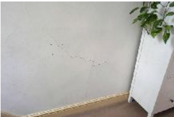
Photo 1 : Basement. Hall refer dwg. no. JGPS/CHAR/4/5/100RevA
