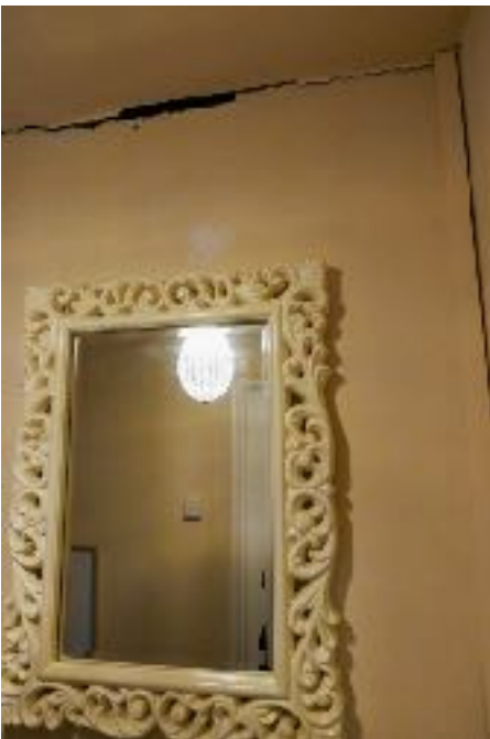
Photo 10 : Second Floor. Refer dwg. nos. JGPS/CHAR/4/5/101RevA, 5016334/RDG/XX/XX/DT/S/0201Rev.T3
