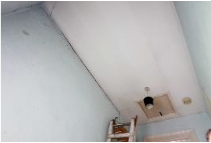
Photo 16: Typical cracks in Second Floor party wall, ceiling and door. Refer dwg. Nos.
