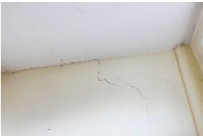
Photo 15: Typical cracks in First Floor party wall.
