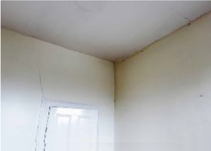
Photo 12: Typical cracks in First Floor party wall and door.
