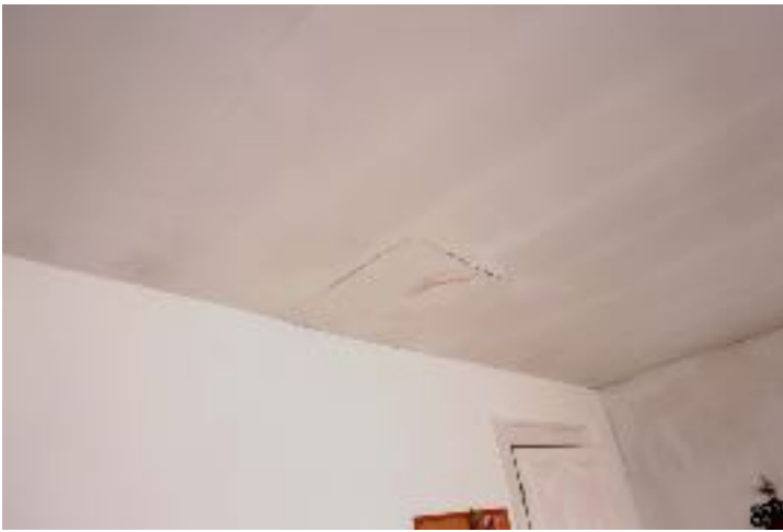
Photo 19: Typical cracks in Second Floor party wall and ceiling.
