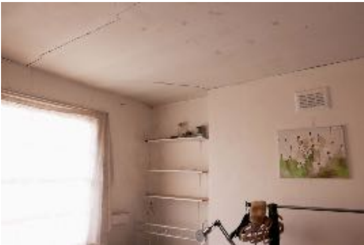
Photo 20: Typical cracks in Second Floor party wall and ceiling.
