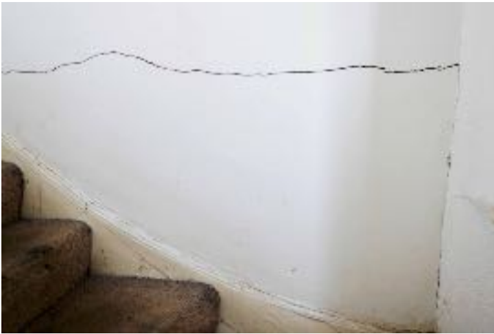
Photo 8: Typical cracks in rear wall on stair landing between first and second floors.
