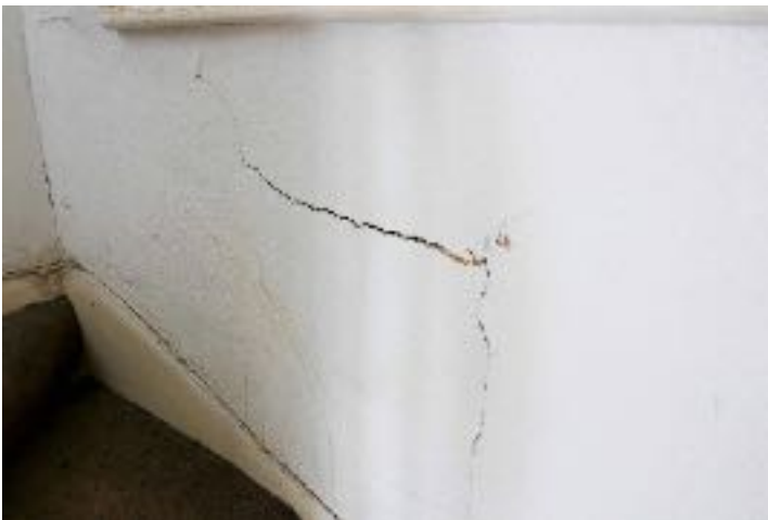
Photo 6: Typical cracks in the rear wall on stair landing between first and second floors.
