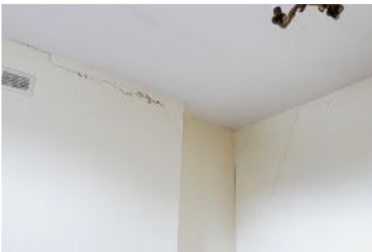
Photo 11: Typical cracks in First Floor rear wall to bathroom.
