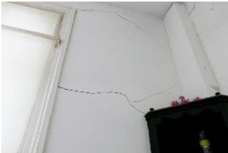
Photo 9: Typical cracks in First Floor rear wall to bathroom.
