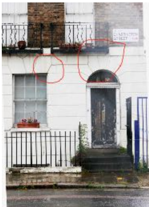
Photo1: Typical cracks in the street front elevation.
