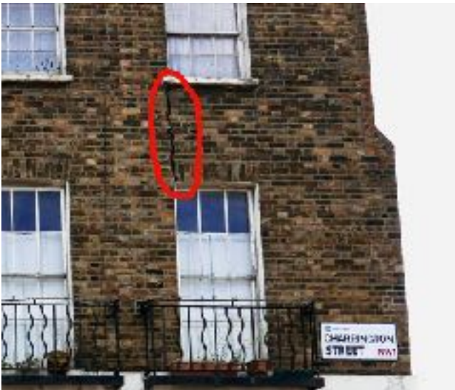
Photo 2: Typical cracks in the street front elevation.
