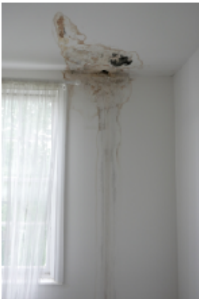
Photo 13 : Second Floor Leak from Attic in bedroom Refer dwg. Nos. JGPS/CHAR/2/3/103RevA
