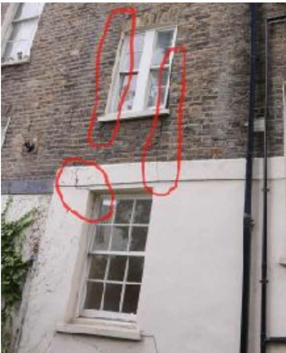
Photo 3: Typical cracks rear elevation
