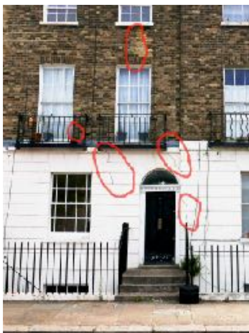
Photo1 : Typical cracks in the street front elevation. Refer dwg. Nos. JGPS/CHAR/2/3/100RevA JGPS/CHAR/2/3/101RevA 5015544/RDG/XX/XX/DT/S/0200/T3 5015544/RDG/XX/XX/DT/S/0300/T3
