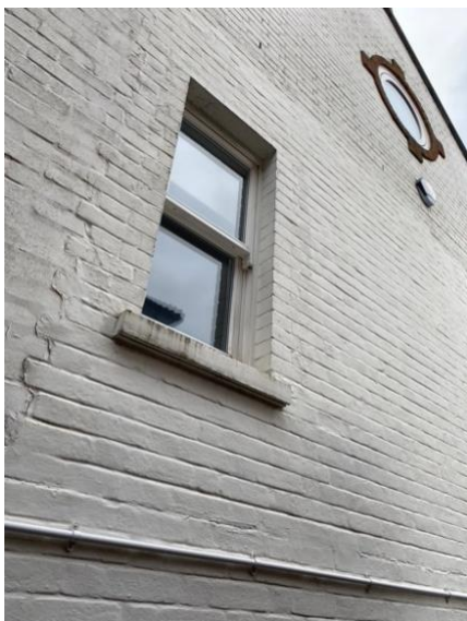
First floor window on South elevation of no.97
