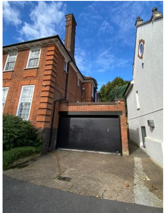
Front drive and existing garage
