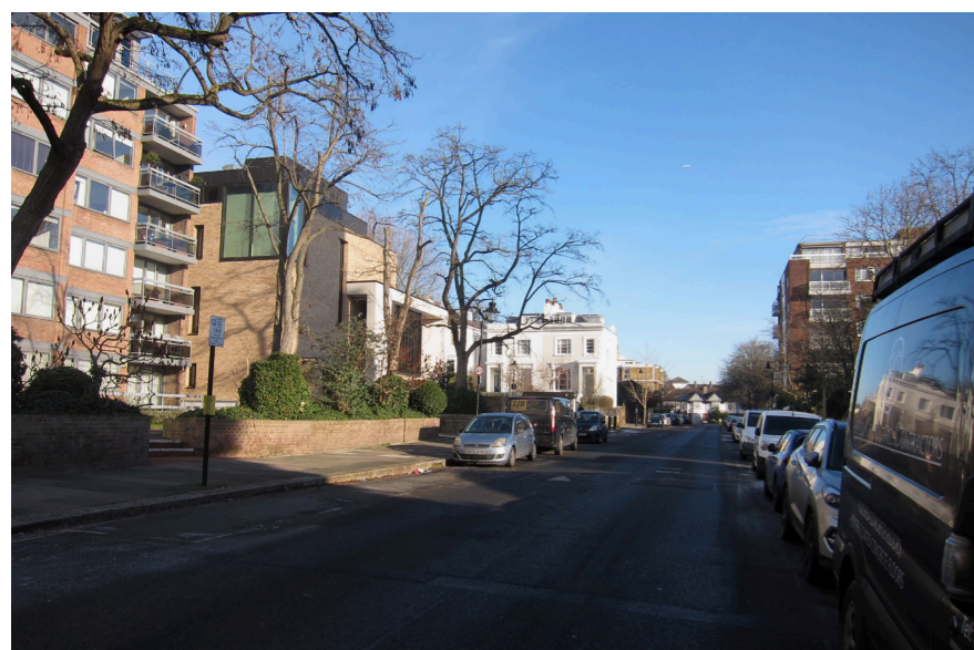
Middle left: View of 13 Eton Villas in context, with neighbours 14-18 Eton Villas stepping up the hill.
