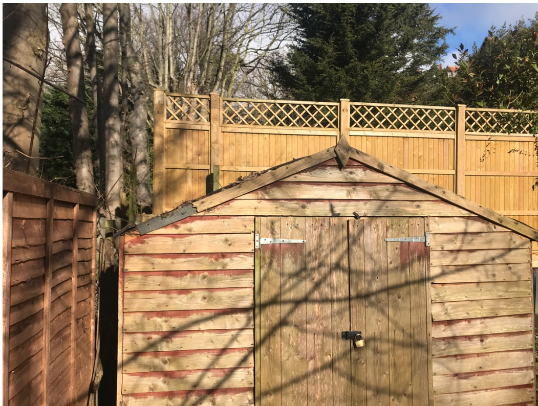
View of the existing garden shed and the rear boundary
