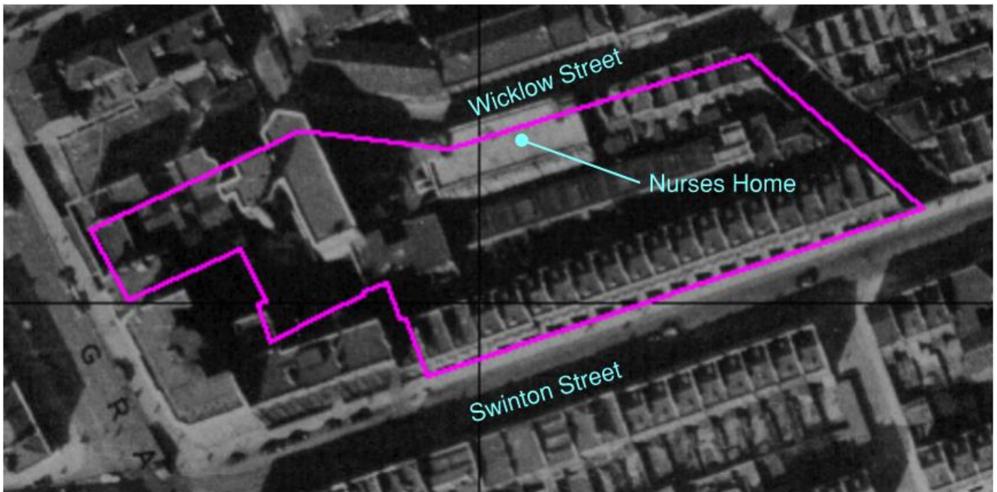
FIGURE 1. Aerial photograph dated 1946 showing the Nurses' Home
