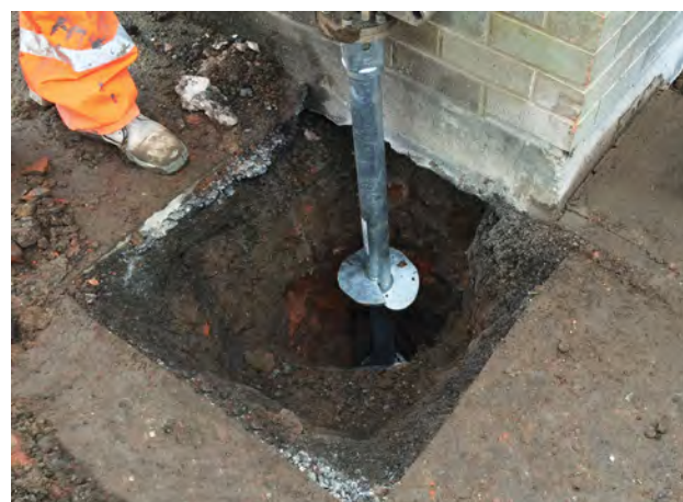
Screw piles can be installed with minimal disruption and digging close to existing buildings.
