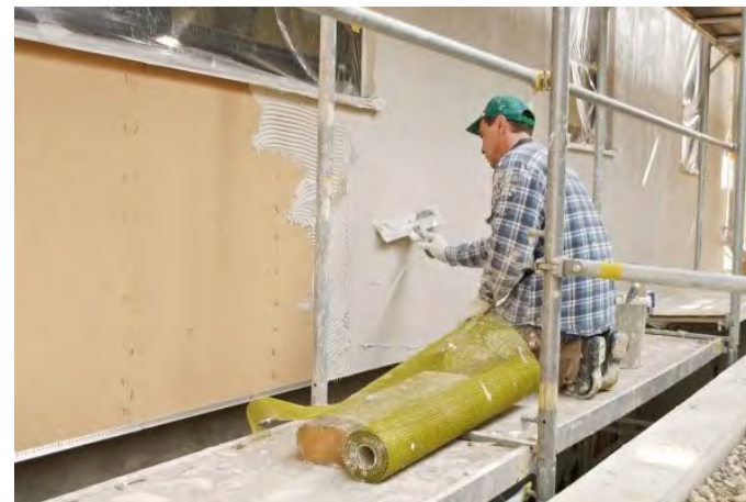
Rendering of wood fibre boards on a building site.
