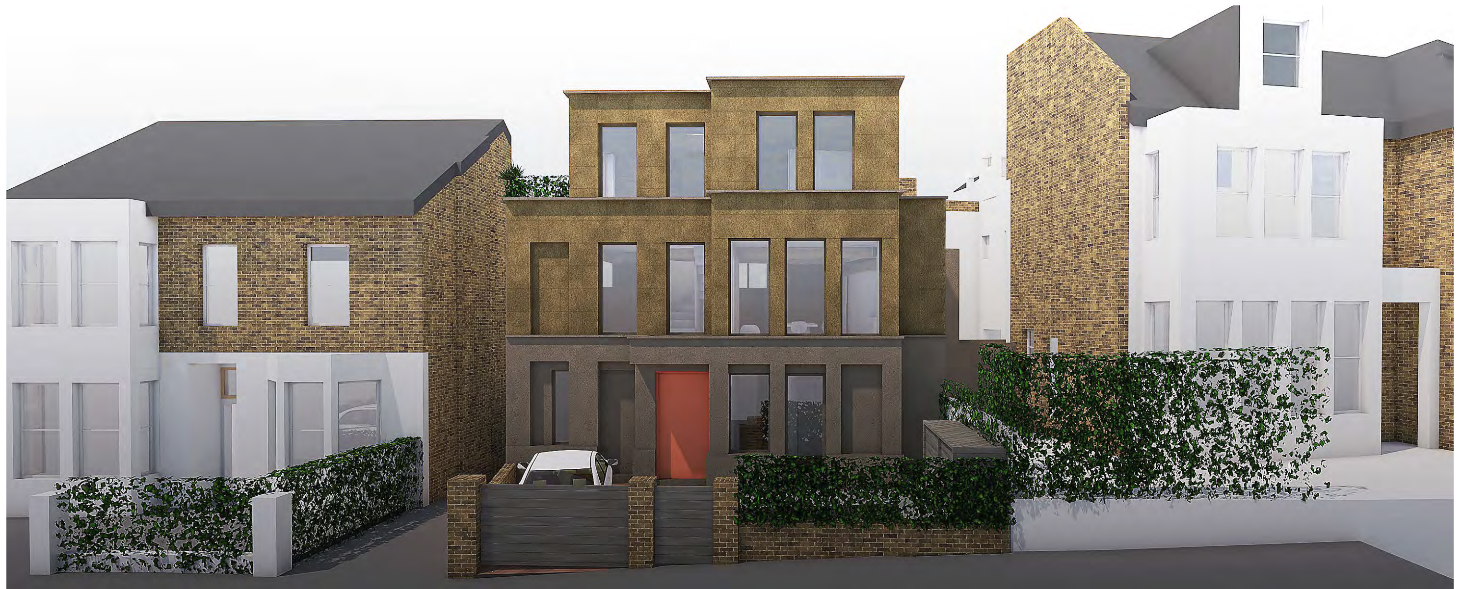
The proposal's front elevation seen in its context. The ground floor is rendered with the upper floors clad in cork. The cork cladding is installed in a stretcher bond pattern with vertical elements around the bay windows.
