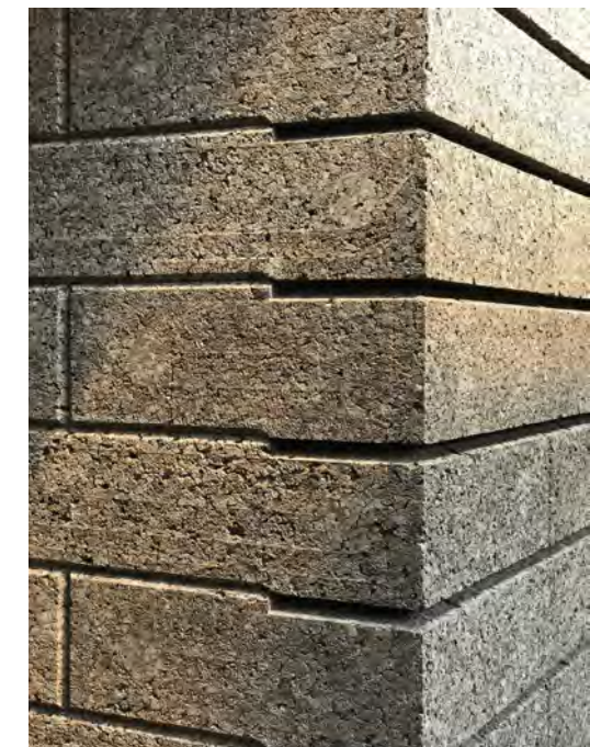
Close up of the cork walls of Cork House (above). Please note that the cork joints have been given a shadow gap to exaggerated separation between elements, which this proposal will not emulate.
