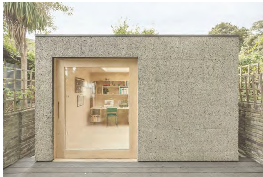
Cork Study - A garden shed in London clad in cork, by Surman Weston Architecture.
