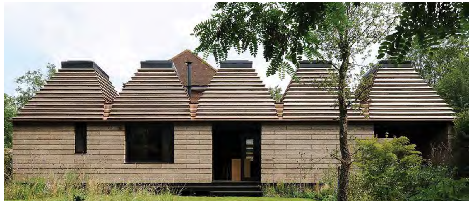
Cork House - A house where the structural walls are made entirely of cork, by Matthew Barnett Howland with Dido Milne and Oliver Wilton
