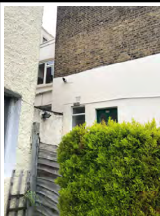
[7] Enclosed wall to north
