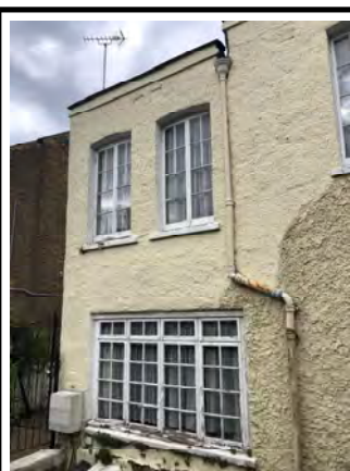
[17] Front facade wall
