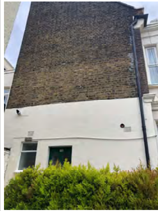
[1] Neighbours wall to north
