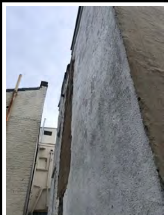
[9] West flank wall
