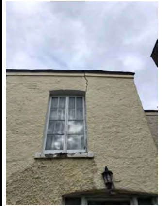
[3] Front facade wall
