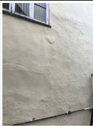
[4] South facade wall
