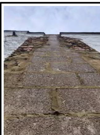
[16] Infilled chimney - west flank wall
