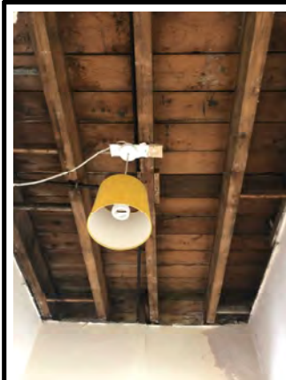
[13] Ceiling over first floor hallway
