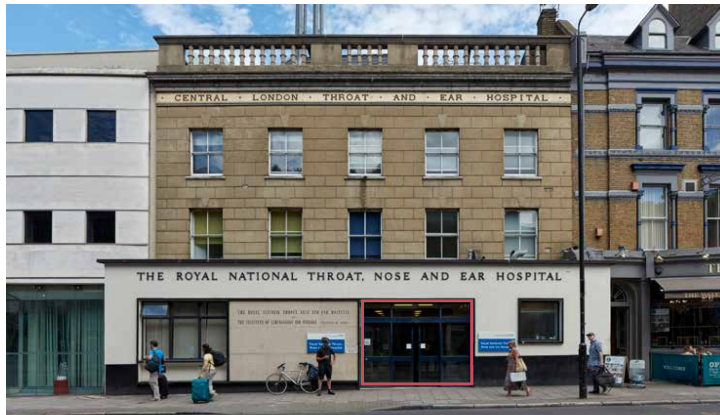
Gray's Inn Rd Retained Facade Affordable Workspace Entrance
