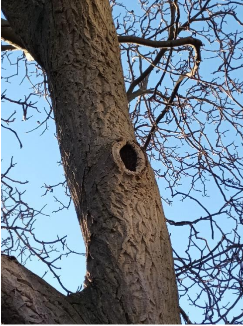
Figure 5: Feature D. Cavity in trunk of mature walnut tree (previously identified and still in the same condition)
