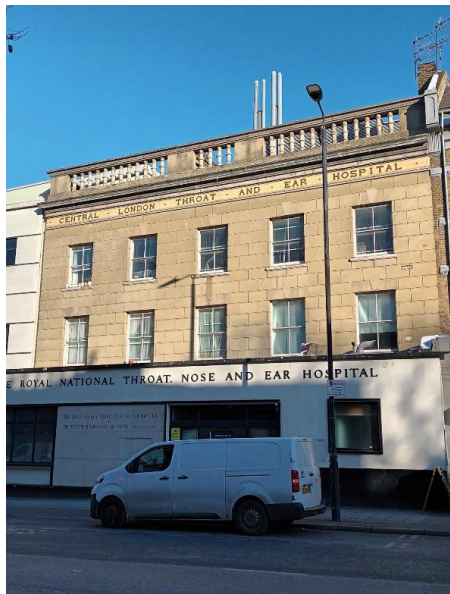
Figure 1: Site entrance on Gray's Inn Road, Western side of the site
