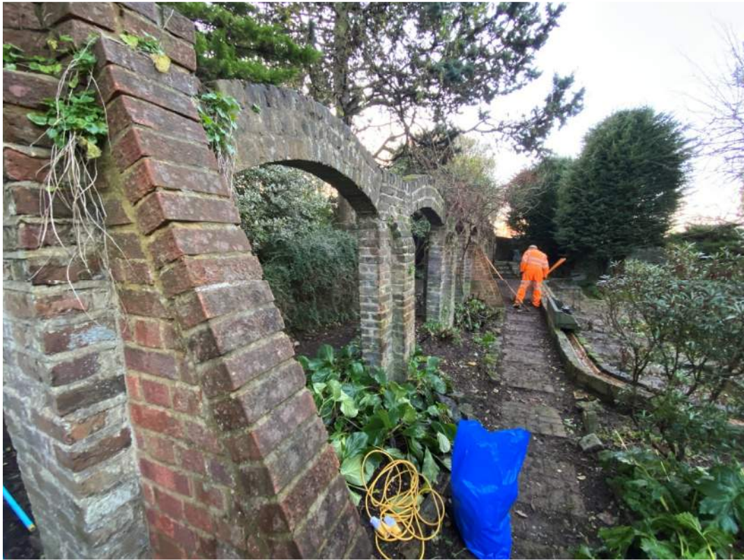
Figure 2 – Existing Arcade and water feature
