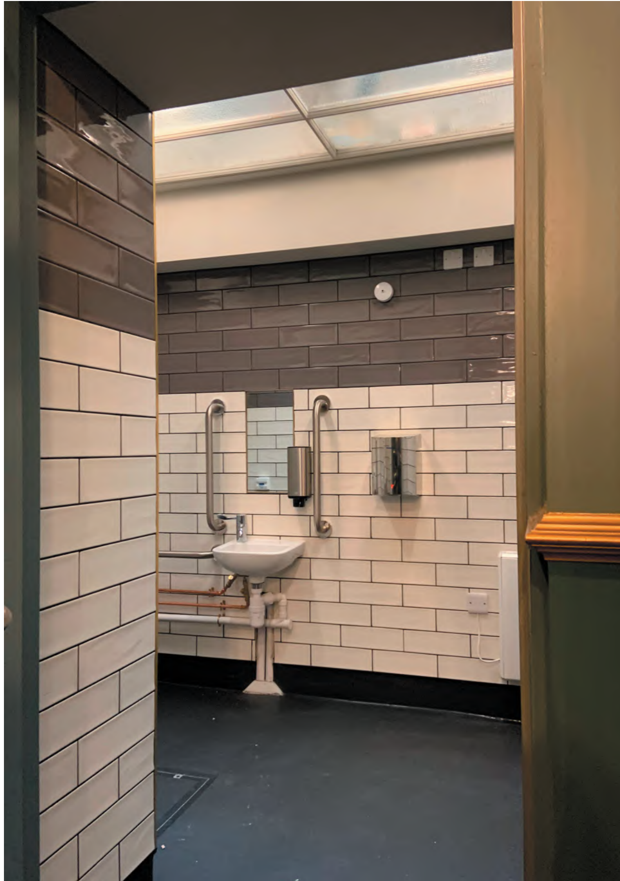
View of the new Acc. WC completed, with the original ceiling glass panels installed
