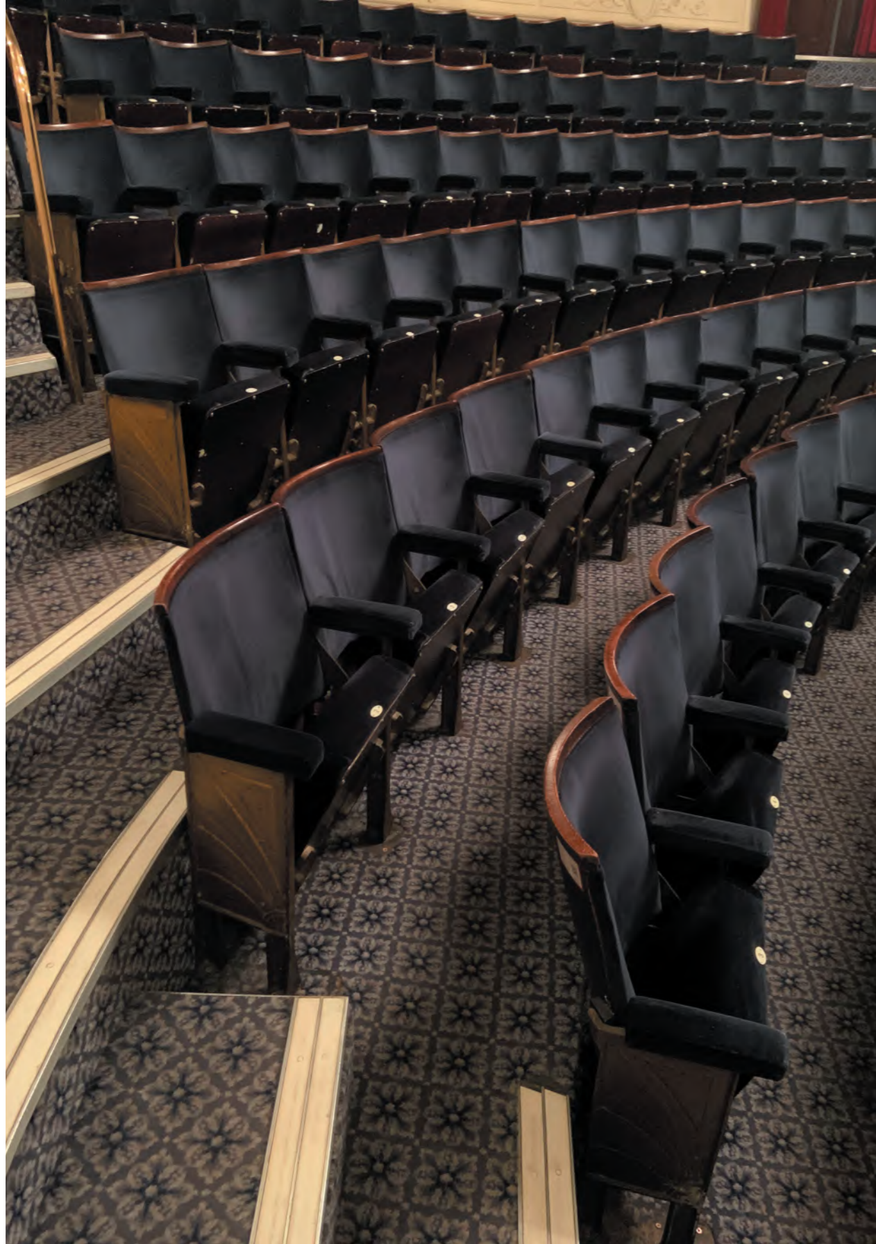
View of the existing seat end panels before the works
