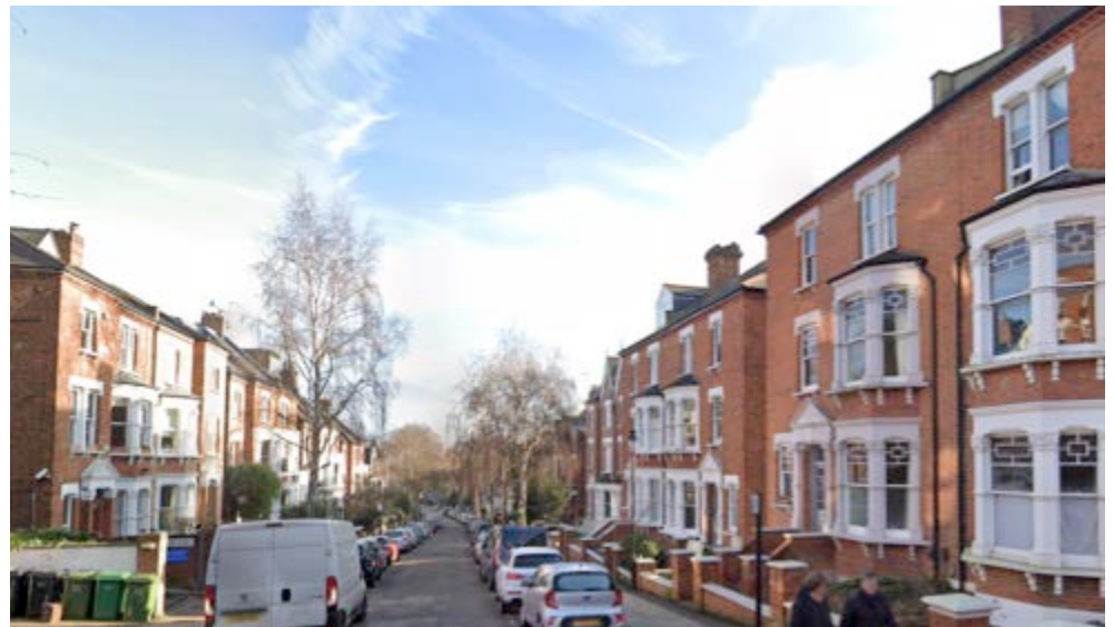
5. Nassington Road, view looking East. Nos 13 & 15 rhs in foreground.
