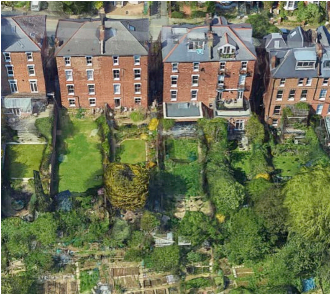
1. Rear elevations No.s 11, 13/15, 17/19, 21/23 (part) Nassington Road
