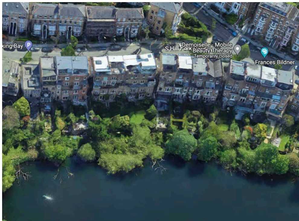
14. Aerial view showing examples of rear extensions to South Hill Park Gardens – visible in public views.
