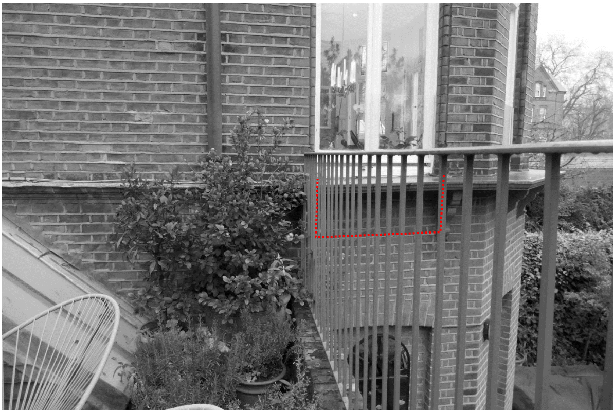
Photo 5: A view of the upper ground floor rear bay window to be changed to a doorway, with the section of proposed removed brickwork highlighted red.
