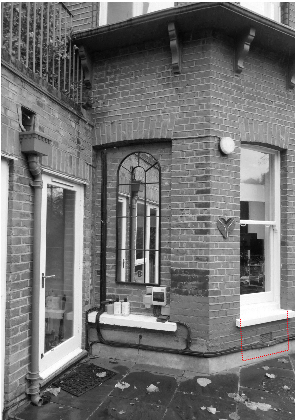
Photo 6: A view of the lower ground floor rear bay window to be changed to a doorway, with the section of proposed removed brickwork highlighted red.
