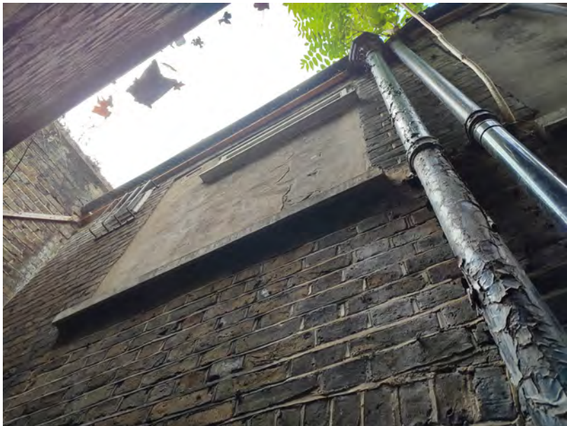
Blocked up ground floor window 1 (from basement courtyard)
