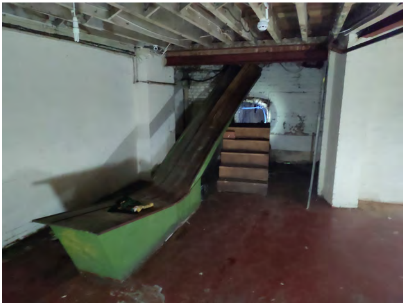
Basement keg/goods ramp, from pavements opening to basement
