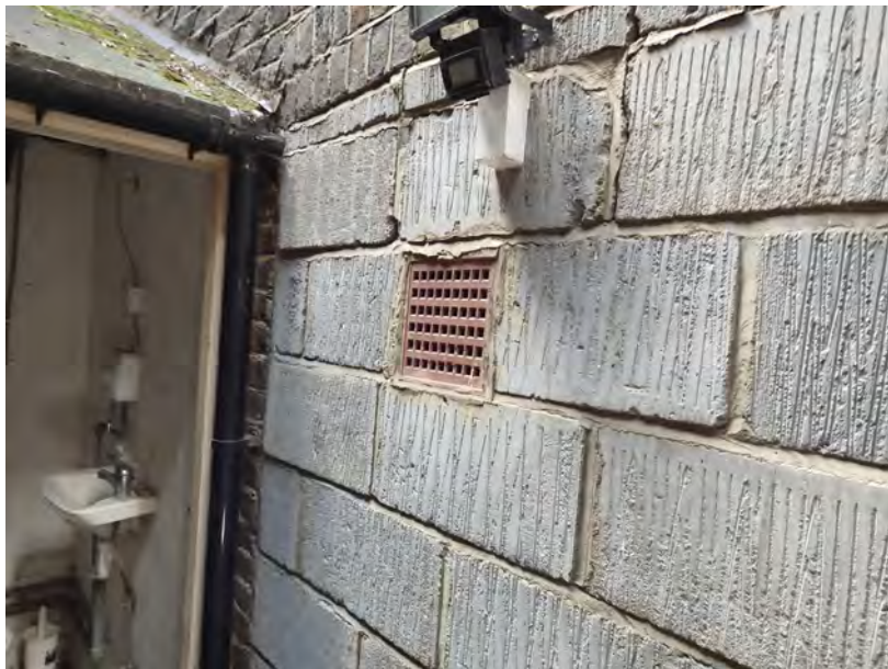
Blocked up basement window from basement courtyard
