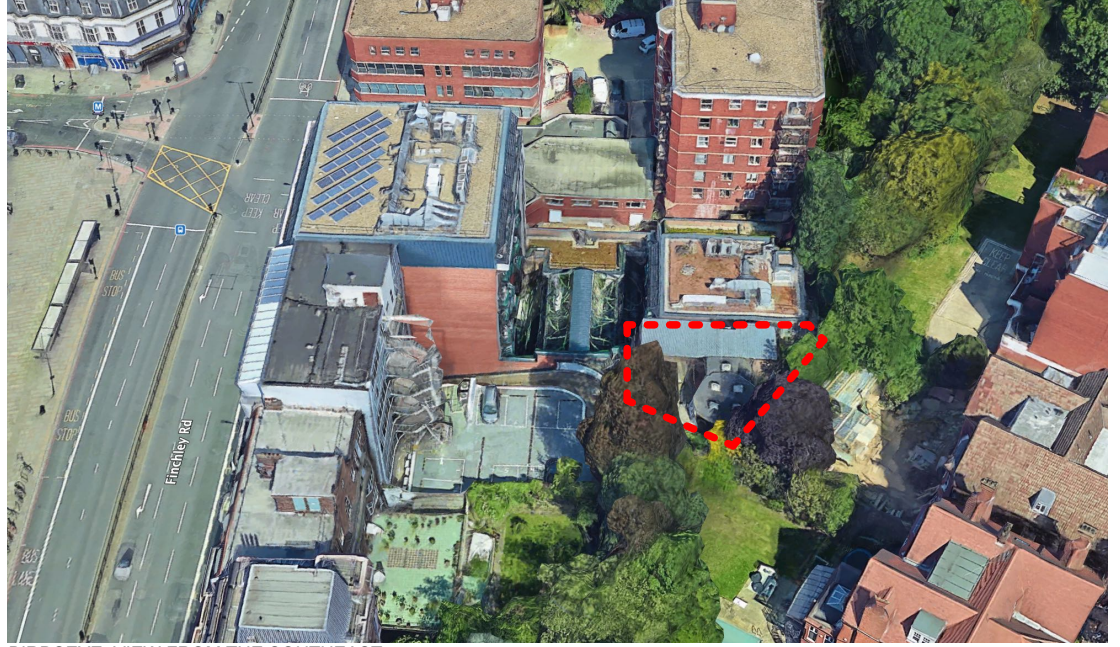
BIRDSEYE VIEW FROM THE SOUTHEAST
