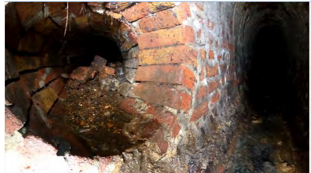
32.00 Connection at 9 o Clock 500mm
