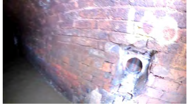
MC1372X_8c0d3c0a-3aed-4716-b126-d2b10da15604_20201211_095136_945.jpg, 00:05:18, 76.00 m Connection other than junction at 3 o'clock, diameter: 100mm, 100mm Con
