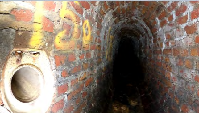
13.50 Connection at 9 o Clock 150mm
