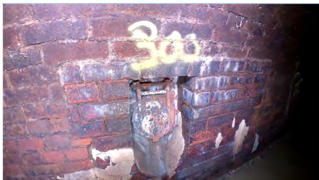
68.00 Connection at 3 o Clock 300mm
