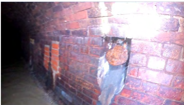
36.00m Connection at 9 o Clock 150mm
