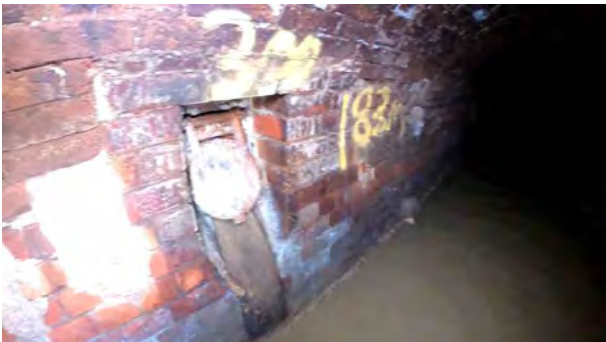
MC1372X_a62d66cd-b0cf-4c23-8340-b6bdc12f9507_20201211_095051_276.jpg, 00:05:38, 82.00 m Connection other than junction at 9 o'clock, diameter: 300mm, 300mm Con
