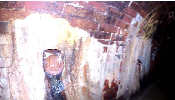
42.00 Connection at 9 o Clock 150mm
