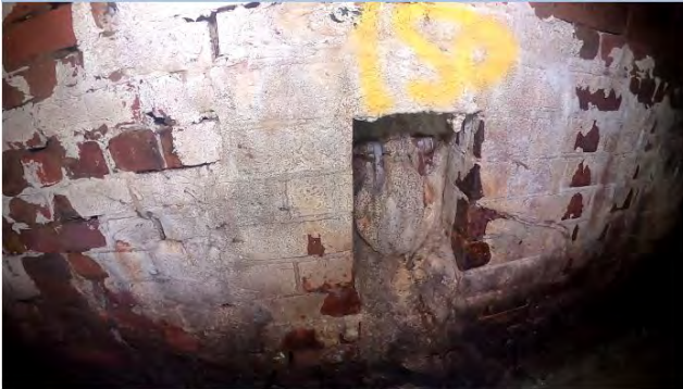
21.00m Connection at 9 o Clock 150mm
