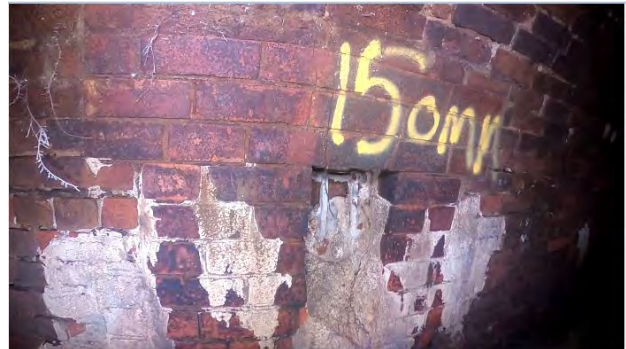
31.00m Connection at 9 o Clock 150mm
