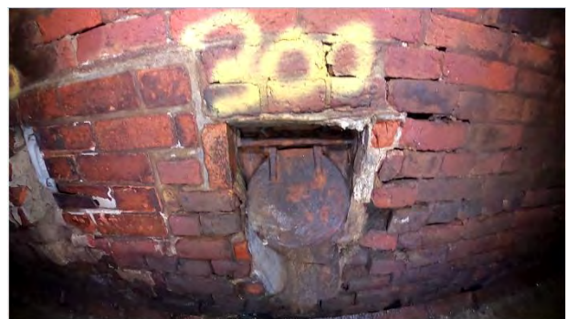
16.00m Connection at 9 o Clock 300mm
