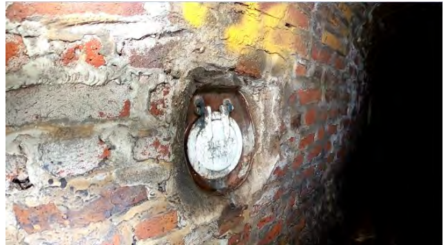
12.50 Connection at 9 o Clock 150mm
