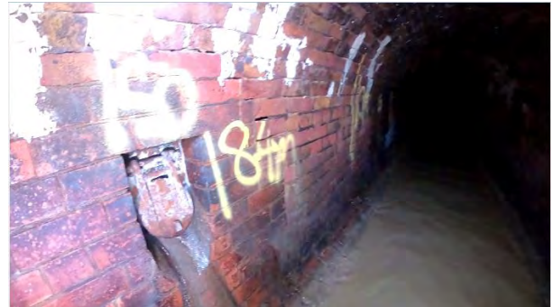
8.40m Connection at 9 o Clock 150mm
