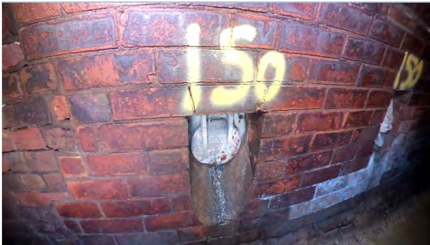
10.00 2xConnection at 9 o Clock 150mm
