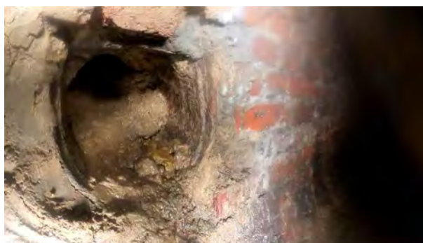
MH4902AX_fefc3b23-0cf1-438b-8c47-fb4c2a833447_20201211_104448_310.jpg, 00:03:58, 42.50 m Connection other than junction at 9 o'clock, diameter: 350mm, 350mm Con
