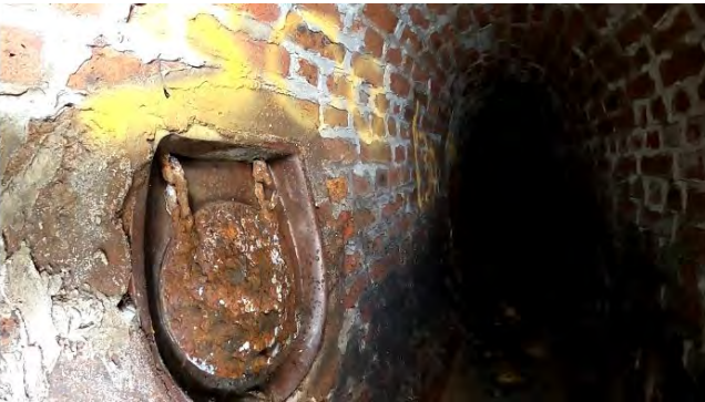
30.00 Connection at 9 o Clock 300mm
