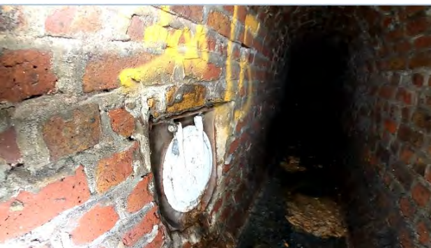
4.50 Connection at 9 o Clock 300mm
