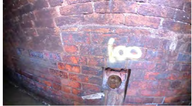
MC1372X_da1af70b-da46-4b46-97f2-af952ad57fbd_20201211_095221_007.jpg, 00:05:02, 72.00 m Connection other than junction at 3 o'clock, diameter: 100mm, 100mm Con
