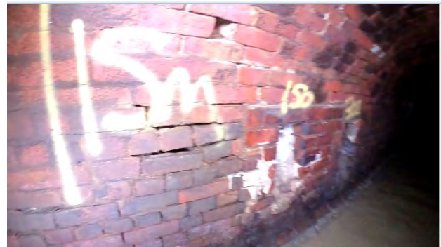
15m Multiple cracks, Mortar Missing
