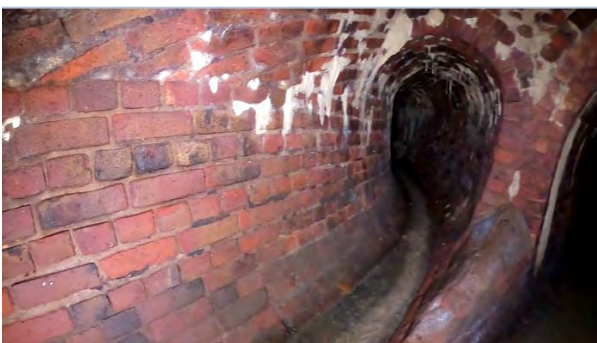
2.50m 1295mm Sewer Connection
