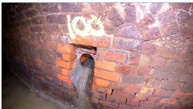
62.00 Connection at 3 o Clock 100mm
