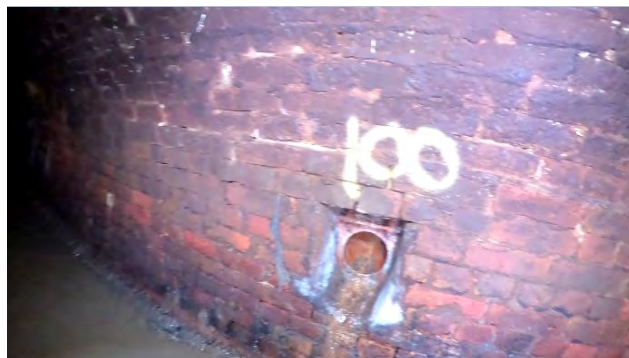
67.00 Connection at 3 o Clock 100mm
