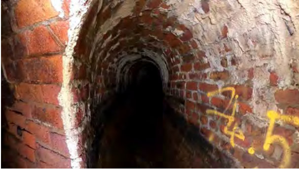
MC1372X_9ccdda8a-0027-49e0-b13b-13d06551b40f_202012 11_095638_393.jpg, 00:00:00, 0.00 m Connection other than junction at 9 o'clock, diameter: 1372mm, Survey Started at Major Connection
