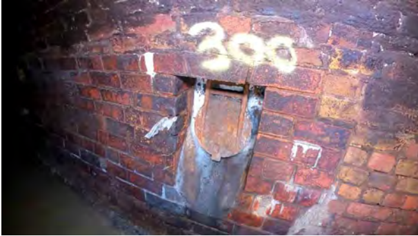
MC1372X_ad6c27c3-8903-491a-ac5f-d8c64a6fac75_20201211_093421_672.jpg, 00:04:54, 70.50 m Connection other than junction at 3 o'clock, diameter: 300mm, 300mm Con
