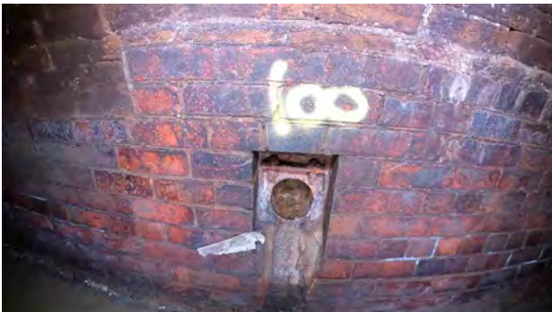
MC1372X_4a48244c-9874-4c19-9f77-3f0de7a4905e_20201211_093458_943.jpg, 00:05:02, 72.00 m Connection other than junction at 3 o'clock, diameter: 100mm, 100mm Con
