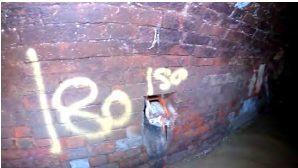
MC1372X_255841da-4d39-4a5b-8d0d-b8e8aa3a0e70_20201211_095120_913.jpg, 00:05:28, 80.50 m Connection other than junction at 9 o'clock, diameter: 150mm, 150mm Con
