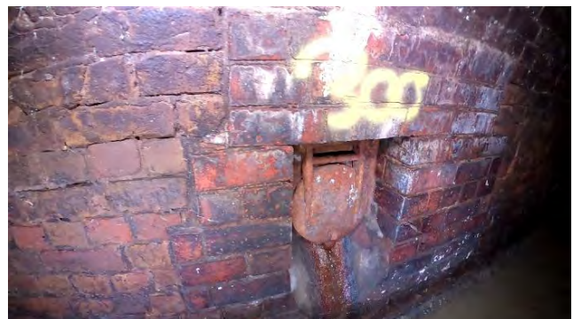
61.00 Connection at 9 o Clock 300mm
