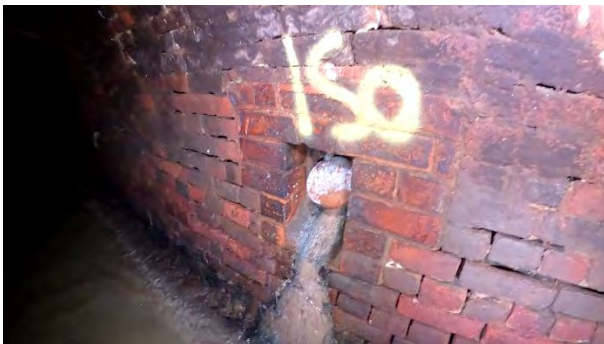
46.00 Connection at 3 o Clock 150mm
