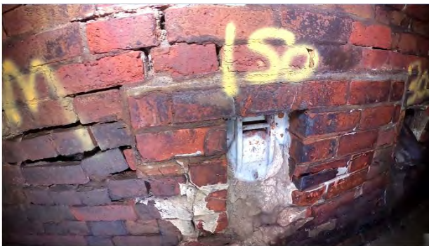
15.50m Connection at 9 o Clock 150mm
