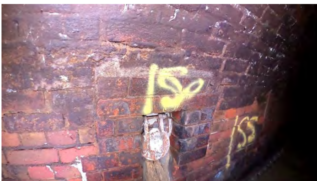
54.00 Connection at 9 o Clock 150mm
