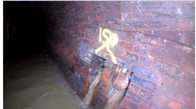
24.00m Connection at 3 o Clock 150mm
