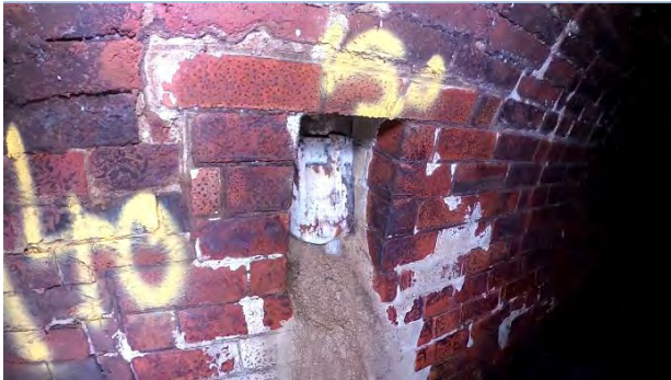
40.50m Connection at 3 o Clock 100mm
