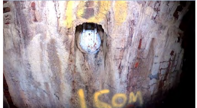
50.00 Connection at 9 o Clock 150mm
