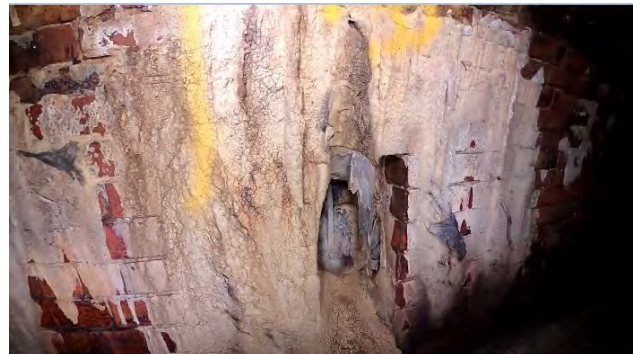
45.00 Connection at 9 o Clock 150mm
