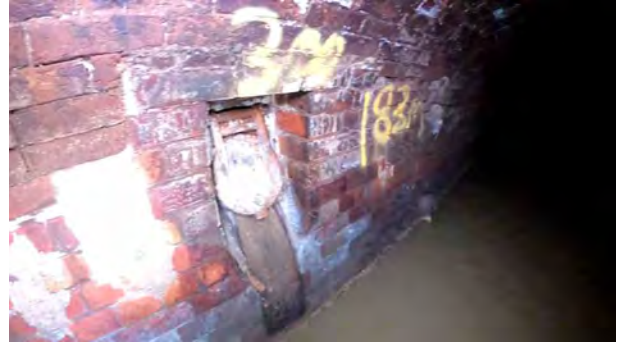
MC1372X_ff0b1625-9f03-48eb-a23b-cea71a467b17_20201211_100206_157.jpg, 00:05:38, 82.00 m Connection other than junction at 9 o'clock, diameter: 300mm, 300mm Con
