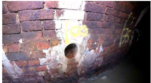
MC1372X_dfd98799-947a-44e5-b673-f282a016c85f_20201211_095145_141.jpg, 00:05:10, 73.50 m Connection other than junction at 9 o'clock, diameter: 100mm, 100mm Con
