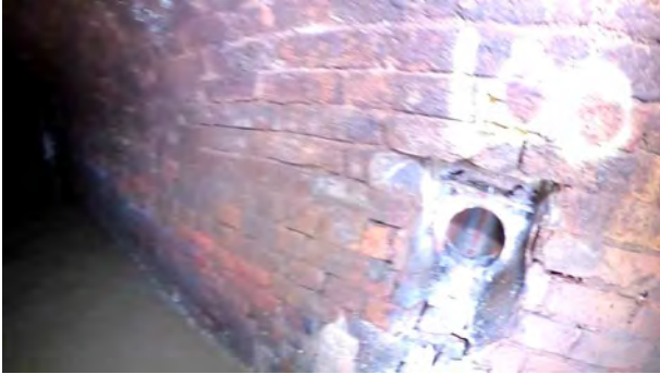
MC1372X_1be12a33-8c6e-482e-826f-43f91534fd60_20201211_095130_087.jpg, 00:05:18, 76.00 m Connection other than junction at 3 o'clock, diameter: 100mm, 100mm Con
