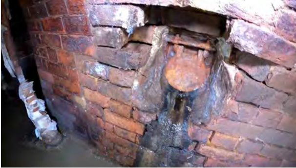
MC1372X_791222b5-4c31-4d7c-aada-64337ead35e7_20201211_095108_447.jpg, 00:05:33, 81.00 m Connection other than junction at 3 o'clock, diameter: 150mm, 150mm Con
