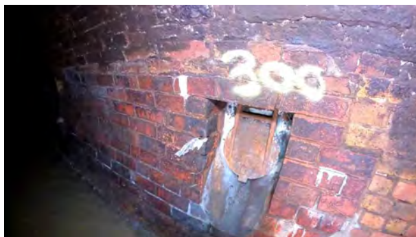
MC1372X_8f797520-370e-4426-9533-694a1b1234c2_202012 11_093350_105.jpg, 00:04:54, 70.50 m Connection other than junction at 3 o'clock, diameter: 300mm, 300mm Con
