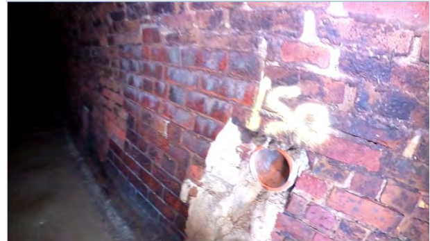
41.00m Connection at 3 o Clock 150mm
