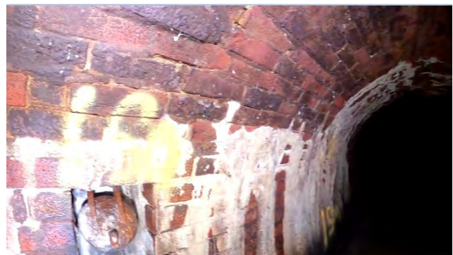
46.50 Connection at 9 o Clock 150mm
