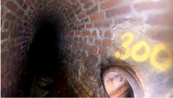
MH4902AX_77eb93a6-188a-40db-958c-24779720c49c_20201 211_104653_141.jpg, 00:04:09, 44.00 m Connection other than junction at 3 o'clock, diameter: 300mm, 300mm Con
