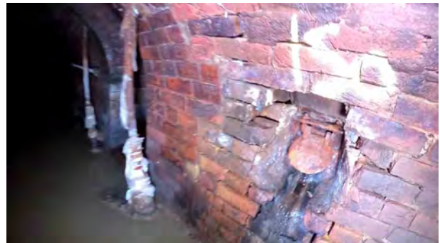
MC1372X_75524d52-5761-4bd6-970a-1e21beacc377_20201211_100236_953.jpg, 00:05:33, 81.00 m Connection other than junction at 3 o'clock, diameter: 150mm, 150mm Con
