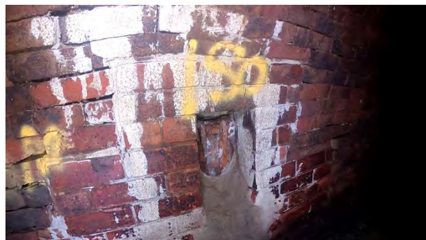
36.50m Connection at 3 o Clock 100mm
