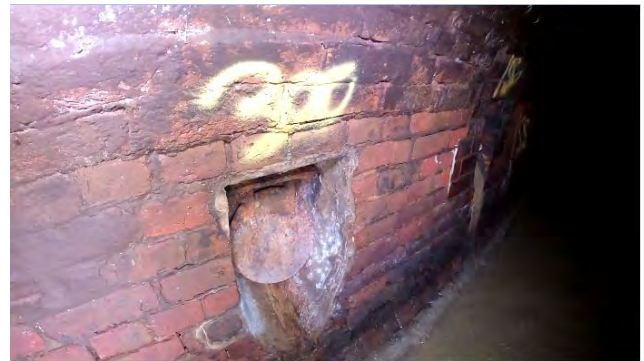
52.00 Connection at 9 o Clock 300mm
