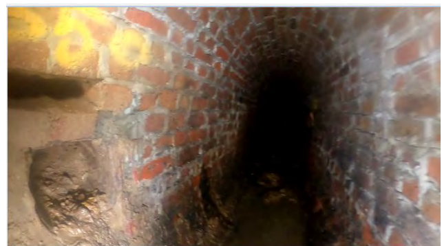
42.50 Connection at 9 o Clock 350mm
