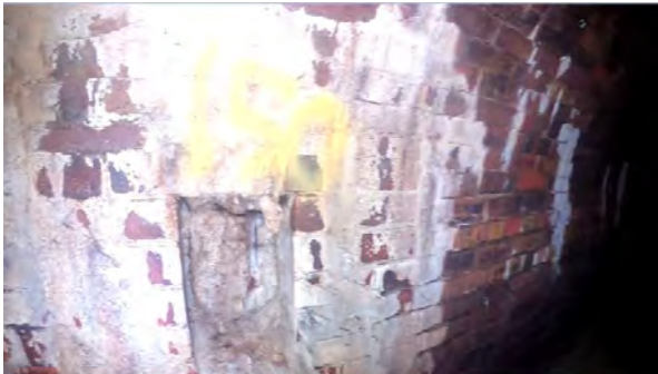
26.00m Connection at 3 o Clock 150mm
