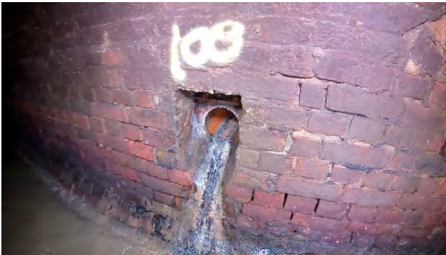
51.00 Connection at 9 o Clock 150mm
