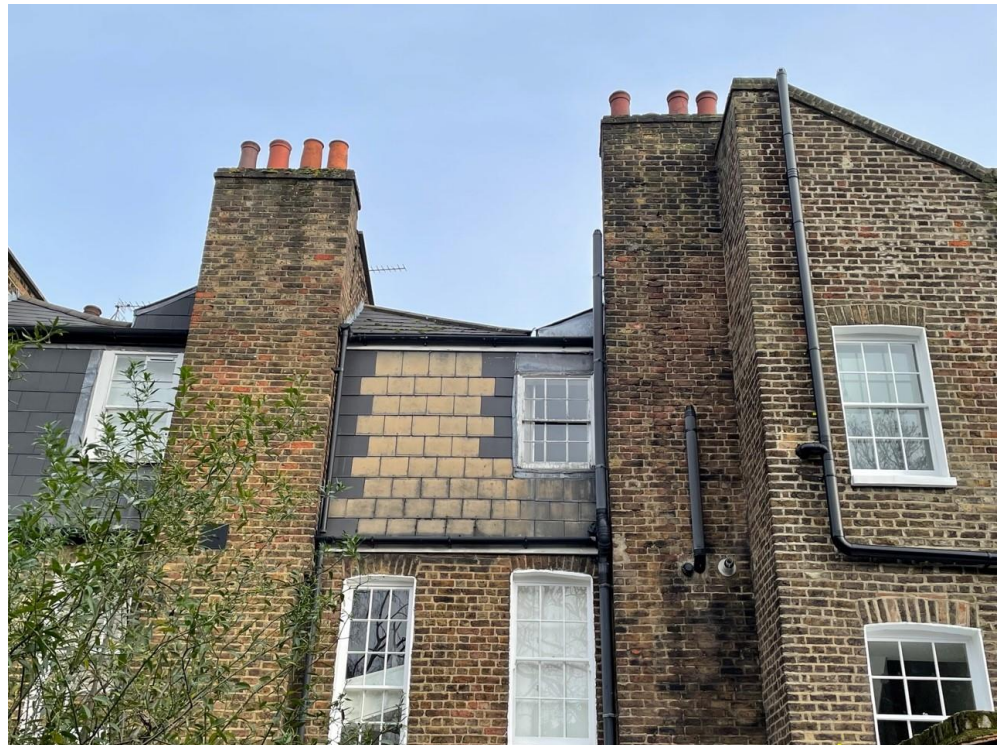
1. View of garden elevation to 135 Arlington Road
