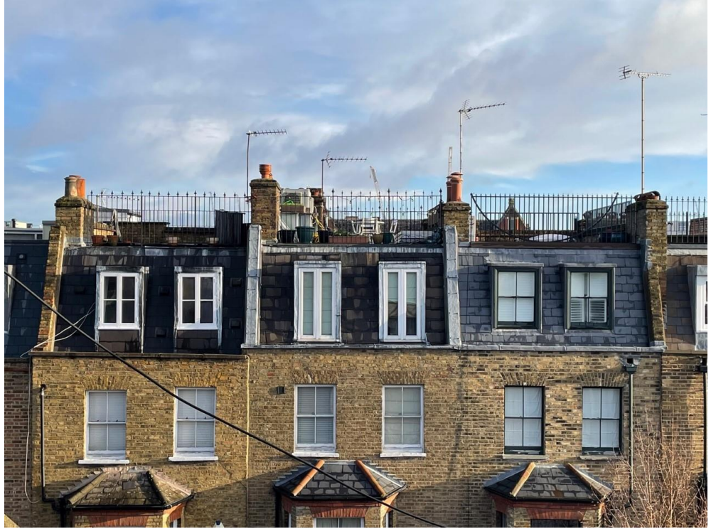
2. View of roof terraces immediately opposite 135 Arlington Road
