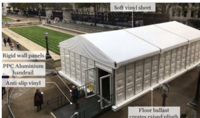
Figure 1 (above): Annotated photo of the external elevations of the structure in the south forecourt
