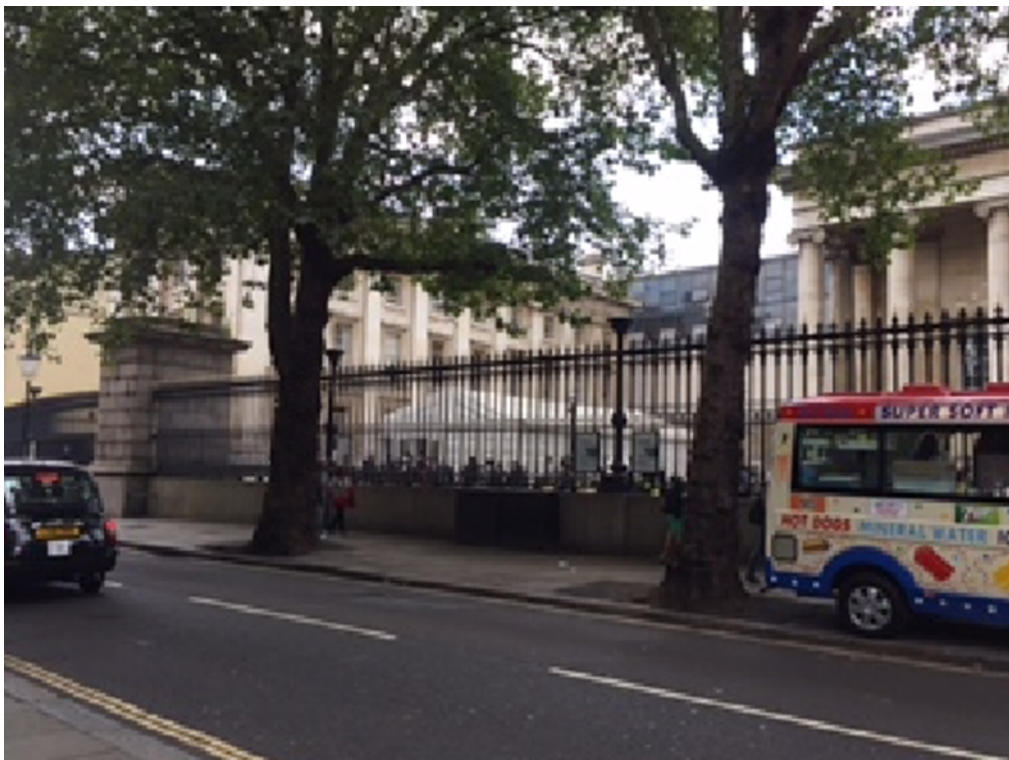
Photo 2 (above): View of security structure in the south courtyard from Great Russell Street
