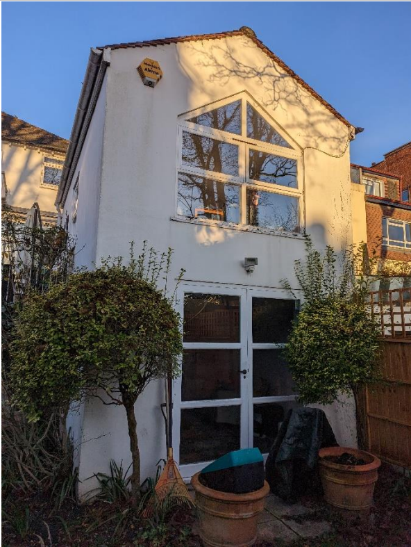
Photo 5 – External Rear wall of ground and lower ground extension
