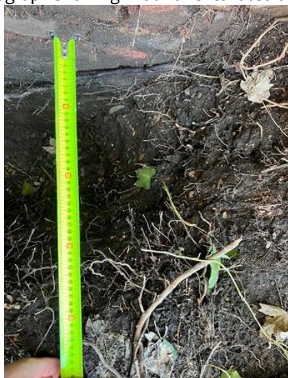
Photograph showing width of excavated trial pit.
