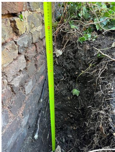
Photograph provided showing depth of top of wall foundation.
