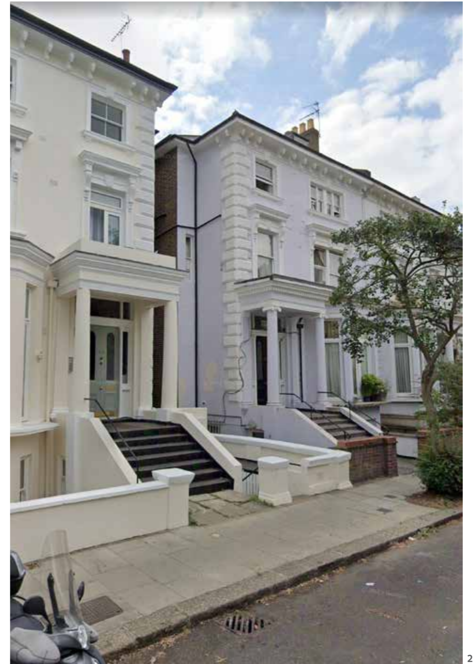
2 Front View of 57 Belsize Park showing adjacent properties
