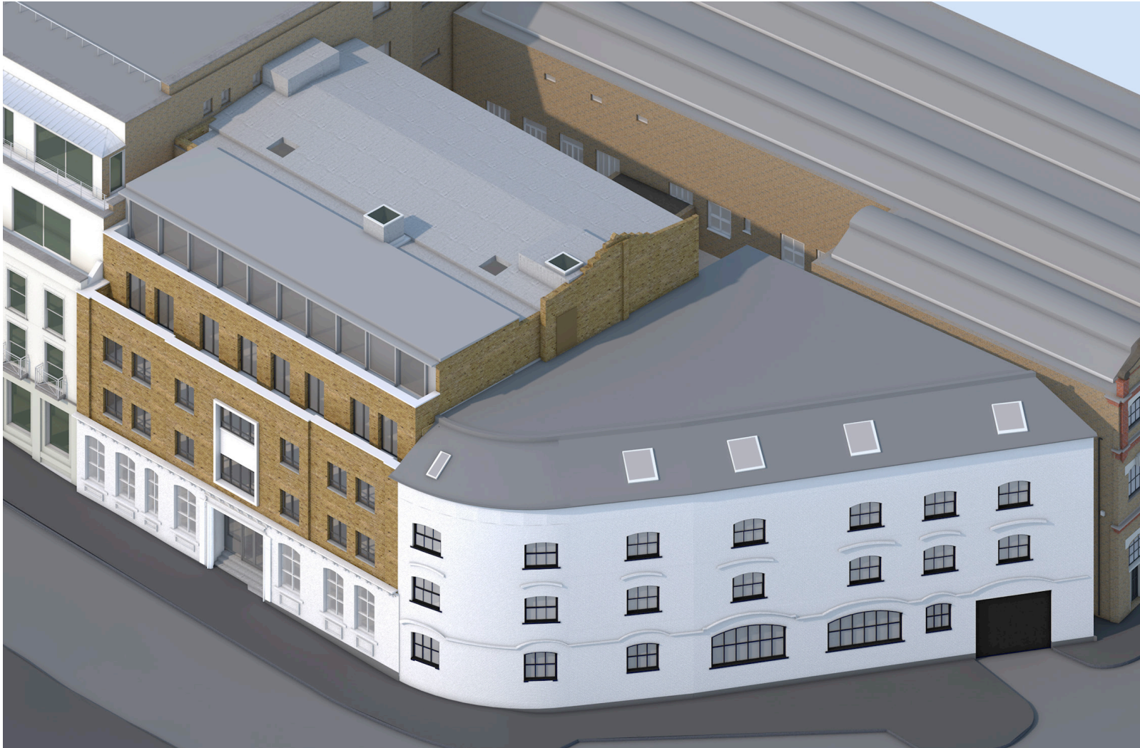
Axonometric ariel view of revised proposal January 2023. The existing building at no. 254 Belsize Road is retained unaltered.
