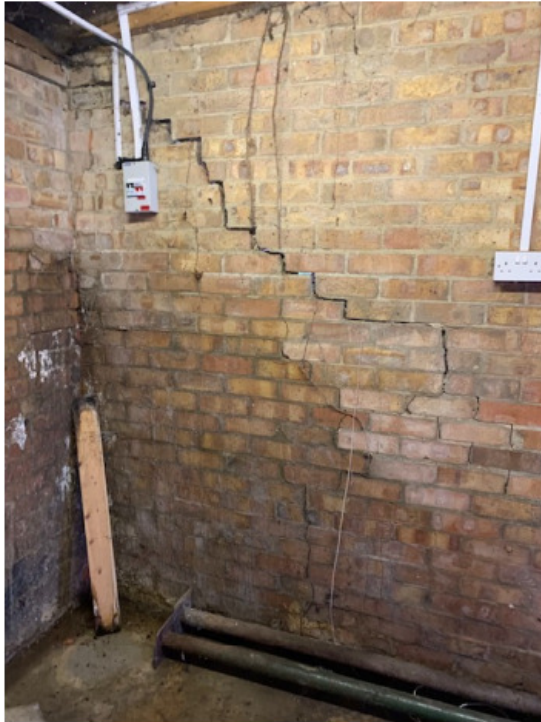
Flank wall of existing garage about to collapse
