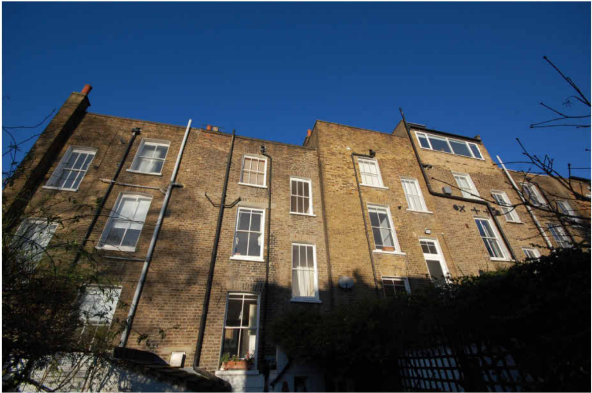
REAR ELEVATION FACING EAST
