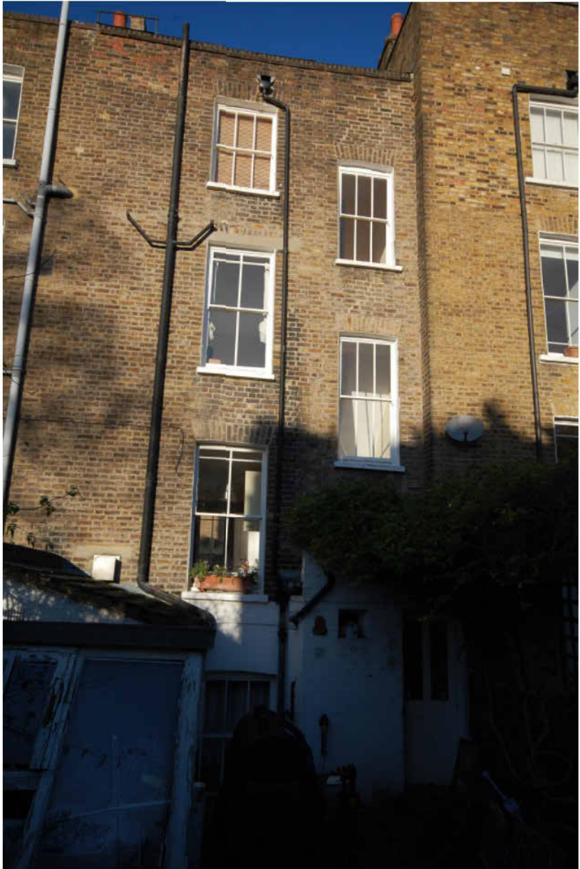
REAR ELEVATION FACING EAST
