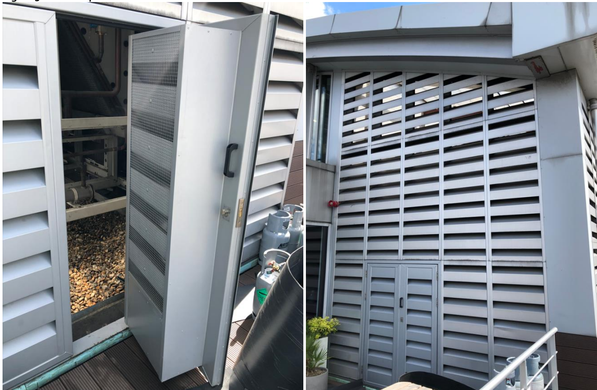
Figure 3.1 Current plant enclosure
