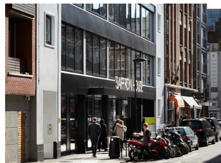
Main entrance on Kirby Street
