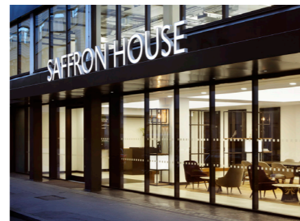
Main entrance on Kirby Street
