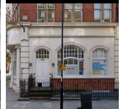
Gated steps - Hastings St.
