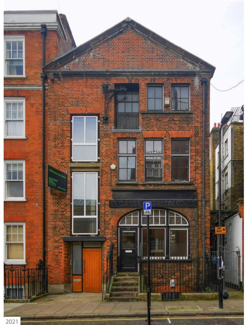
Fig. 19. Current exterior view of 73-75 Kenton Street
