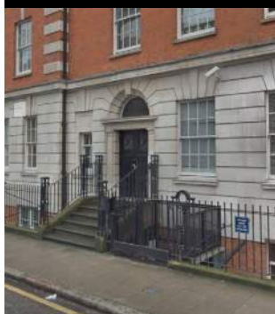
Lightwell lift - Bidborough St.
