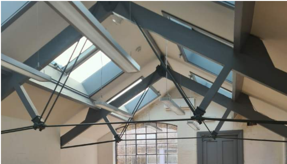
Fig. 24. Second floor - Roof Skylights and Timber Fink Truss Roof
