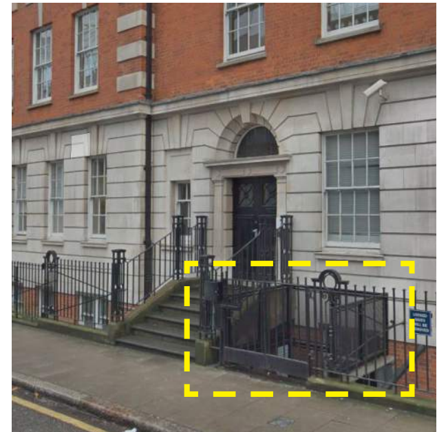
Fig. 16. 38 Bidborough Street with external platform lift
