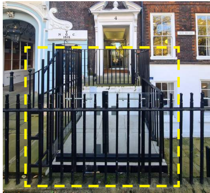
Fig. 15. 1 New Square with external platform lift
