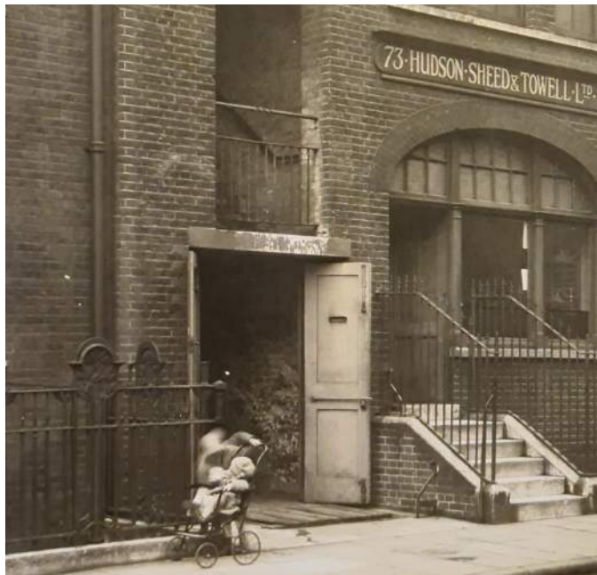
Fig. 8. Original Door at 73-75 Kenton Street
