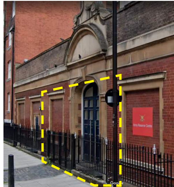
Fig. 9. Army Reserve Centre, with concrete plinths and metal swing gates
