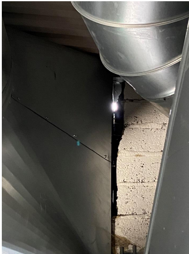
Photo 4: Small gap in wall next to ventilation tunnel
